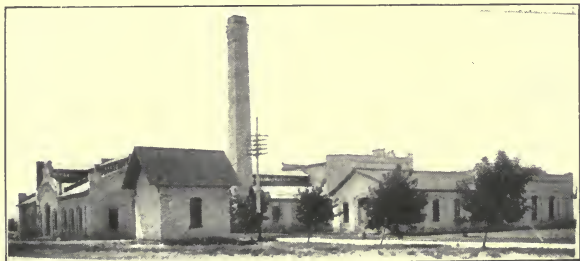
Rear View of Mechanic Arts Buildings.
