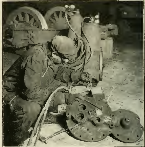
Welding 8½-In. Cross Compound Air Compressor Head
