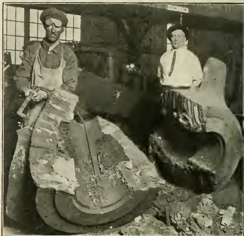
Fig. 6—Cast-Iron Propeller Hub After Being Cut by Oxyacetylene Cutting Torch
