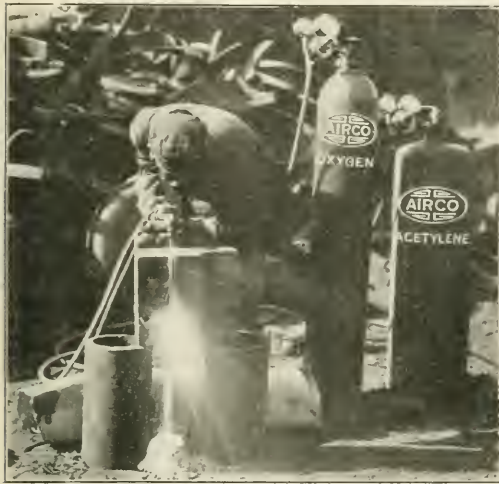
Fig. 2—Cutting 14-In Steel. Very Little Smoke
