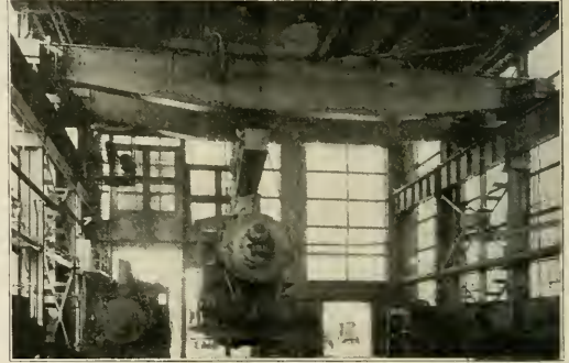
Lifting the Locomotive from the Longitudinal Track
