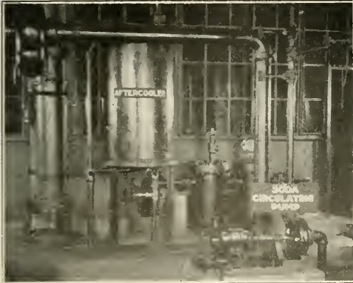
Fig. 4—Aftercooler for Reducing Temperature of Compressed Air
