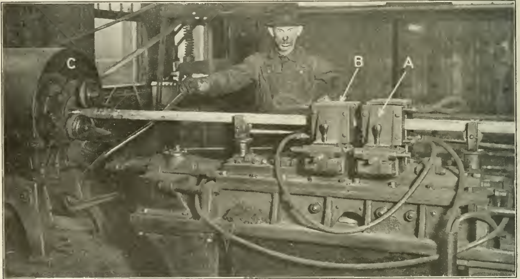
Fig. 1—Rolling a Boiler Tube After It Has Been Safe Ended in Thomson Electric Butt Welder
