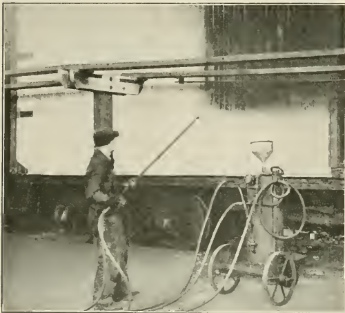
Fig. 1—Operation of Paint Spraying a Box Car
