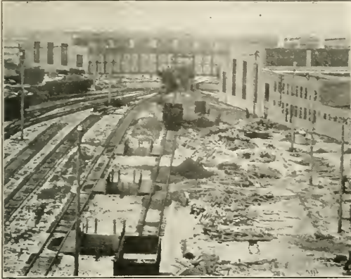
Arrangement of the Three Ashpits on Inbound Tracks
