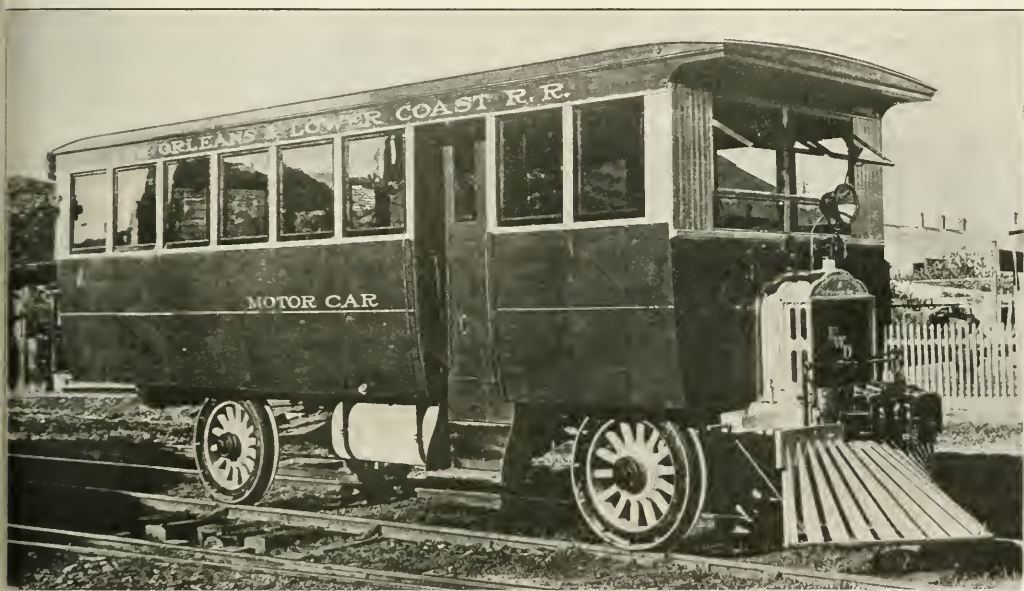
Four-Wheel Drive Rail Car Used on a Sixty-Mile Run Between New Orleans and Buras
