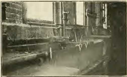
Fig. 1—Vats and Drying Coil for Cleaning Triple Valves with Caustic Soda
