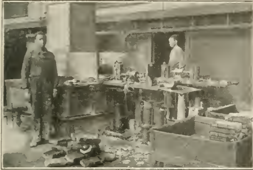
Fig. 2—Equipment for Relining Car Journal Brasses
