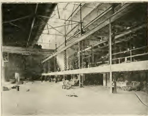
Fig. 2.—Battery of Electric Carbide Furnaces at Modern Plant of National Carbide Corporation
