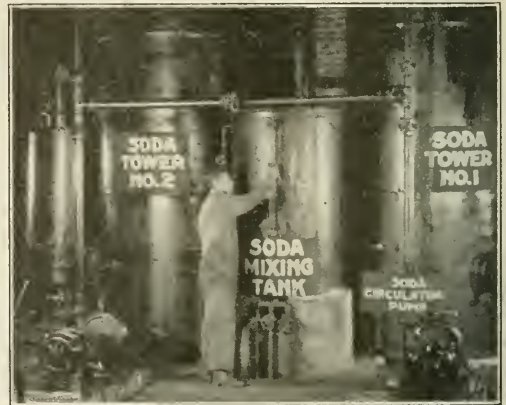
Fig. 3—Towers for Removing Carbon Dioxide from Air Oxygen
