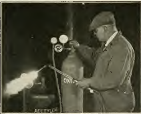
Fig. 1.—Burning Acetylene Before Compressed Oxygen Is Supplied
