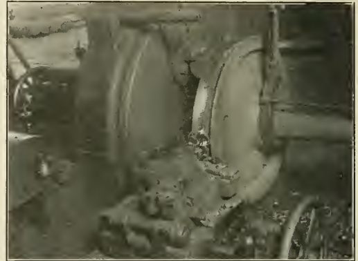
Fig. 3—No. 18A Roughing Tool Used in Sellers Car Wheel Lathe
