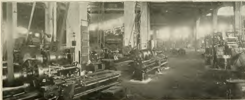
An Interior View Showing the Crane Bay
