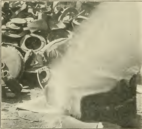
Fig. 1.—Cutting Through 12 Inches of Cast Iron
