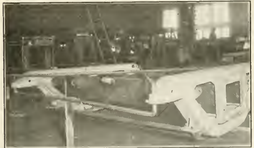
Trams for Squaring Tender Trucks While Assembling
