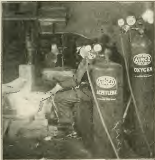
Improvised Preheating Furnace for Cast Iron Welding
