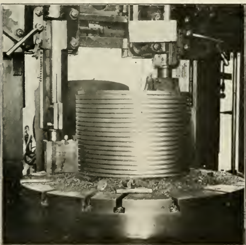
Fig. 1—Boring Inside Surface of Packing Tub Automatically Severs the Finished Packing Rings
