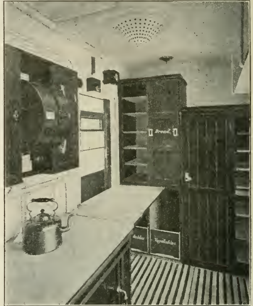
View of Kitchen, Showing Change-Over Switch and Cupboard.
