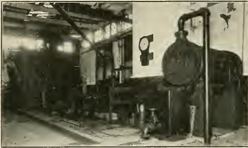
Fig. 1—The Test Plant, Showing Boiler (at left), Booster and Condenser
