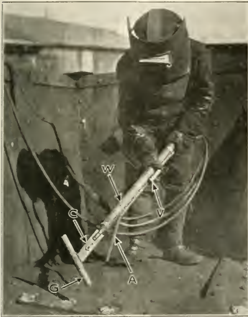
Fig. 2—Burning Tool in Use on a Flat Surface
