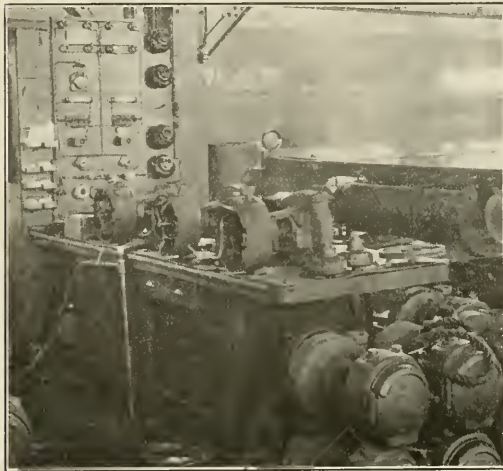
Fig. 3—Bench and Test Rack for Pyle-National Generator Sets
