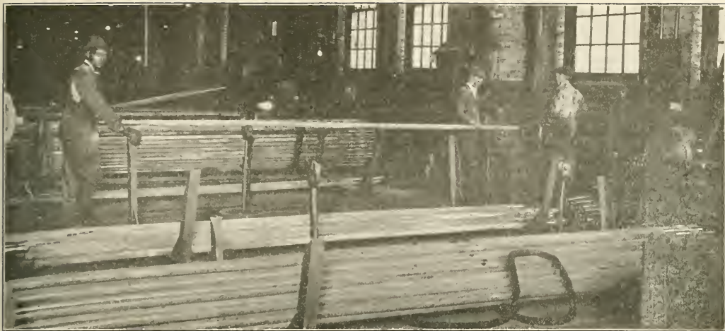
Fig. 1—View of Well Organized Flue Shop
