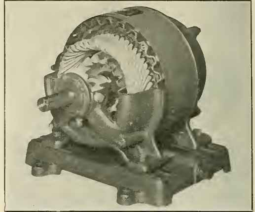
Ventilating Air is Reversed to Keep Oil Out of the Windings
