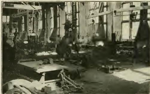
General View of P. & L. E. Blacksmith Shop at McKees Rocks
