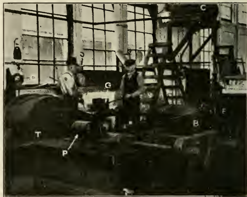
Fig. 1—Spring Tester and Gage with Furnace and Oil Bath in the Background
