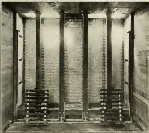
View of Bunker Before Bulkhead is Applied, Showing Removable Ice Grates
