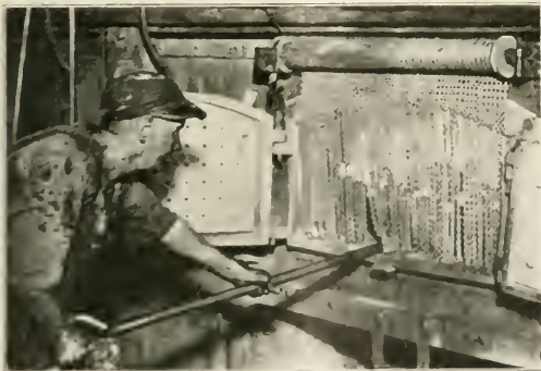
Cleaning a Fire Through a Wiegand Chain Screen Door
