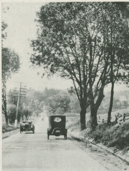
Trees must be far enough from the edge of the pavement to permit adequate drainage, and to allow future widening of the road if increased traffic makes it necessary.
