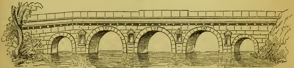
BRIDGE AT ARIMINUM.
