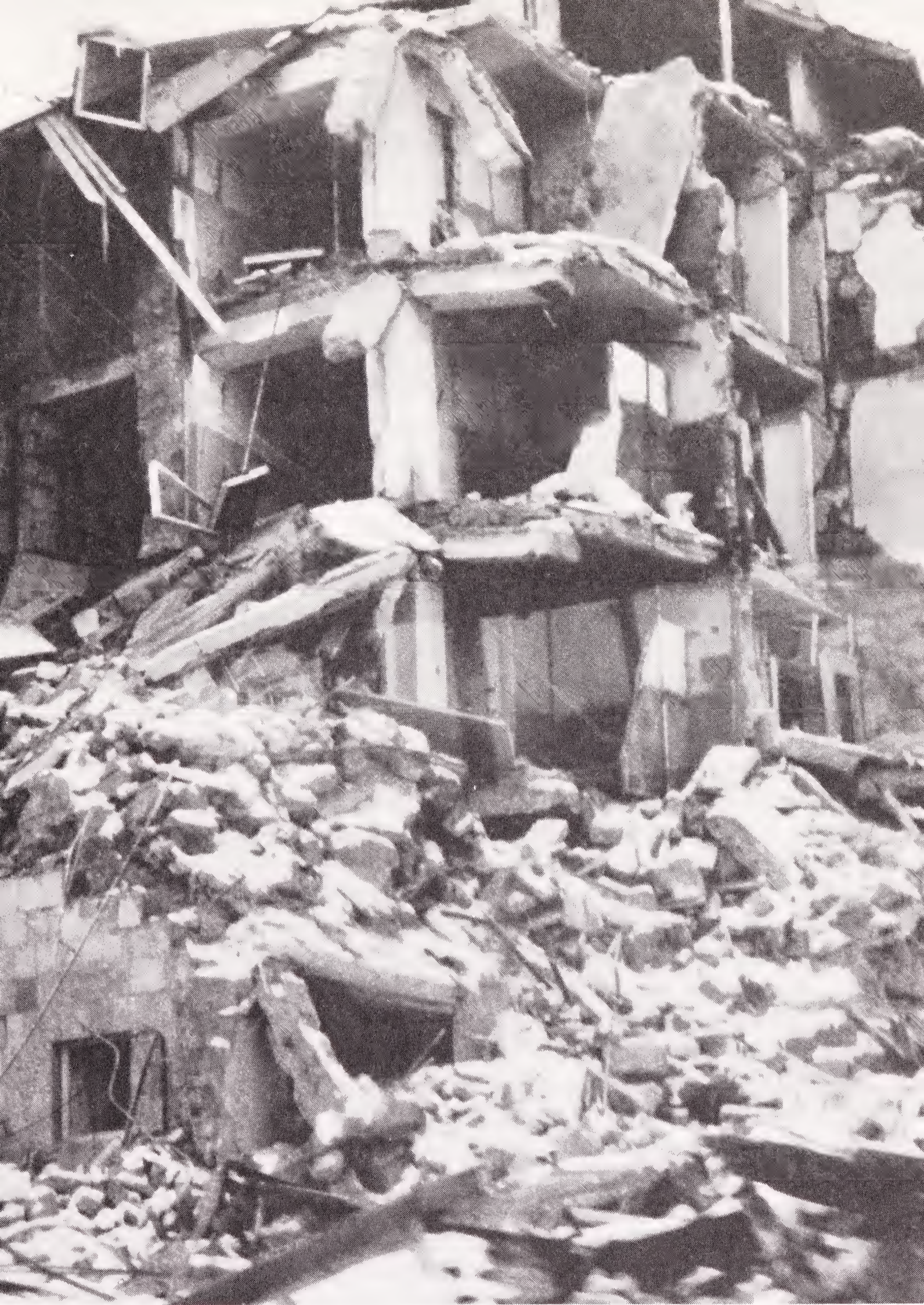
Apartment house in Spitak, Armenian Republic, destroyed by an earthquake in December 1988 that registered 6.9 on the Richter scale. Such apartment houses were not designed, or built, to withstand seismic activity of that magnitude. The earthquake claimed 25,000 victims. Courtesy United States Geological Survey
