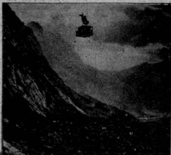
An Aerial Cableway.
