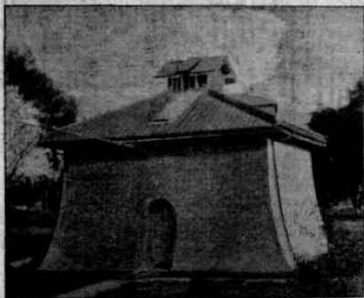
AN EARTHQUAKE-PROOF BUILDING, Erected in the grounds of the Imperial University, Tokyo.
