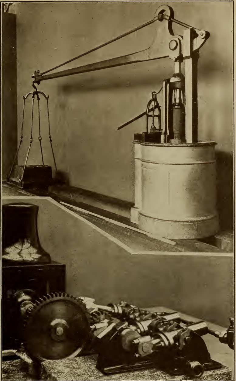
HYDRAULIC PRESS AND HYDRAULIC CAPSTAN.
