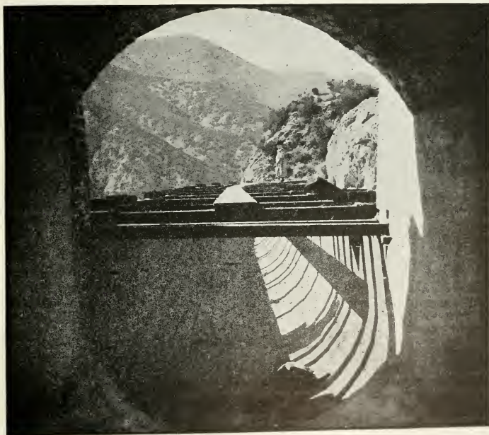
CONNECTION BETWEEN TUNNEL AND FLUME OF SANTA ANA CANAL, CALIFORNIA.
