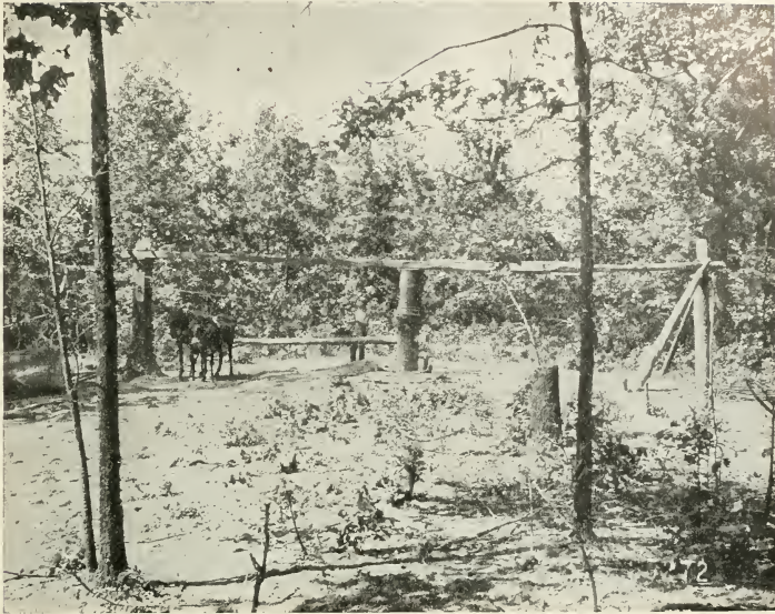
DRUM FOR DRAWING LOGS FROM COVE TO THE PLATEAU, SEWANEE.
