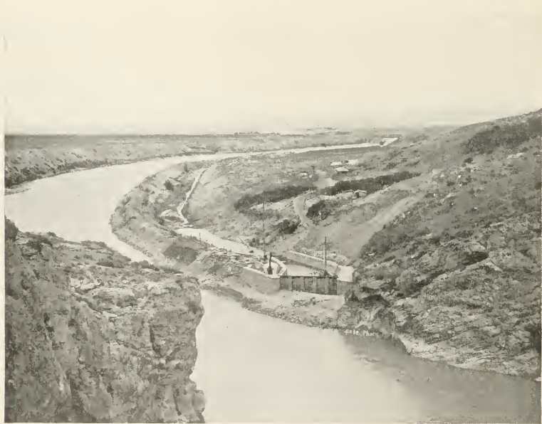
Photo by D. S. Cole, Hot Springs, S. D. HEADGATE AND PART OF CANAL, BIGHORN RIVER, MONTANA. THIS CANAL ON THE CROW RESERVATION IS THE LARGEST AND MOST IMPORTANT OF THE INDIAN IRRIGATION WORKS NOW UNDER WAY.
