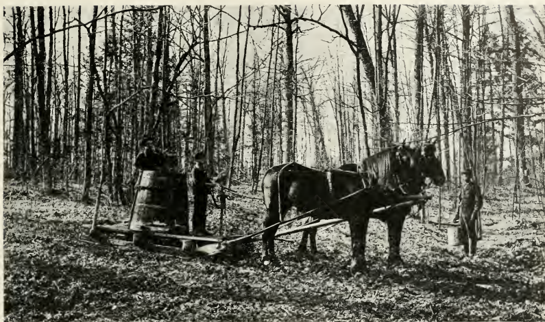
THE GATHERING TANK, WYOMING COUNTY, PA.
