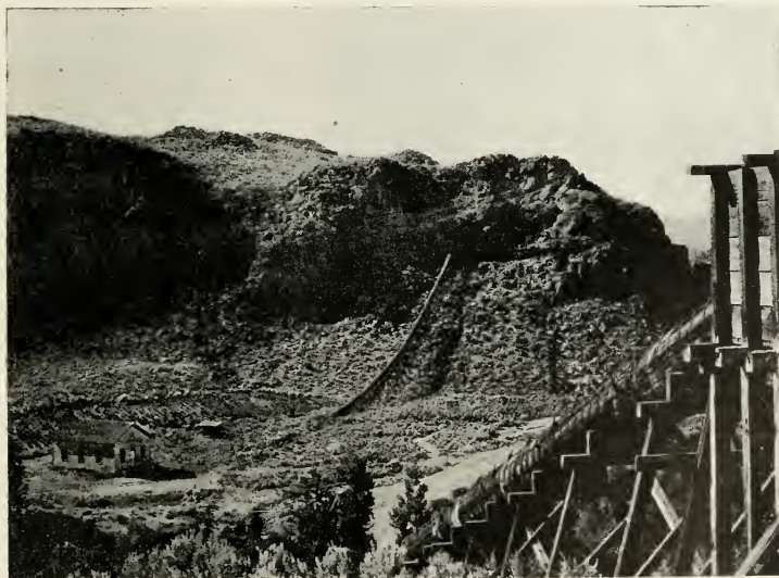
INVERTED SIPHON OF THE YAKIMA VALLEY CANAL COMPANY, NORTH YAKIMA, WASHINGTON.
