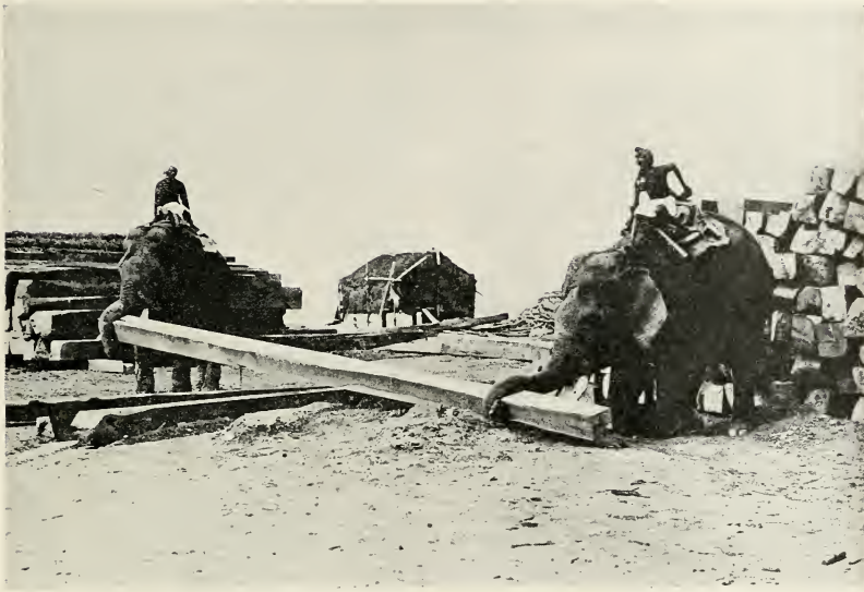
ARRANGING TEAK IN A LUMBER YARD.
