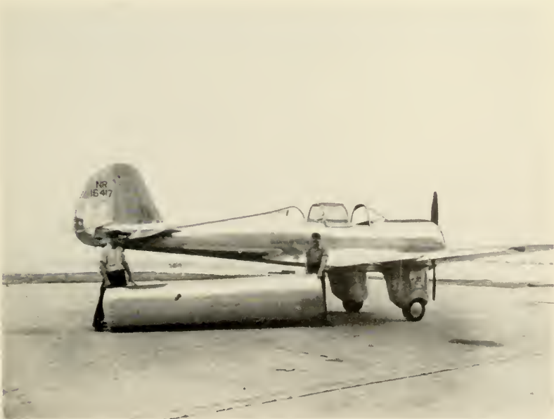
2. CURTISS-WRIGHT MODEL 20. Fuel tank size comparison.
