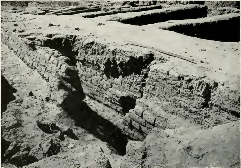
1. Foundations of the larger (and inner) of the two outer fortification walls, with the glacis built against it. The foundations of the perpendicular main wall were deeper than those of the sloping glacis, which was bonded into the main wall about six or seven rows of bricks above its base.
