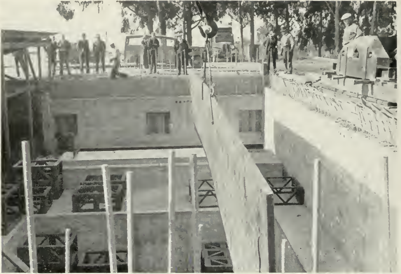
1. The first base plate being placed on the concrete foundation. The plate is 52 feet long, 75 inches wide, and 2 inches thick, and weighs 13\frac{1}{2} tons. There is about 1,200 tons of reinforced concrete in the foundation.
