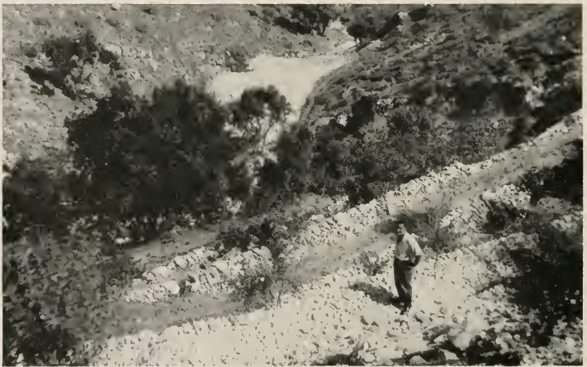
2. NEWLY BUILT TERRACES WHICH ACT AS SIEVES FOR WINTER STREAMS AND THUS COLLECT A THIN LAYER OF SOIL.
