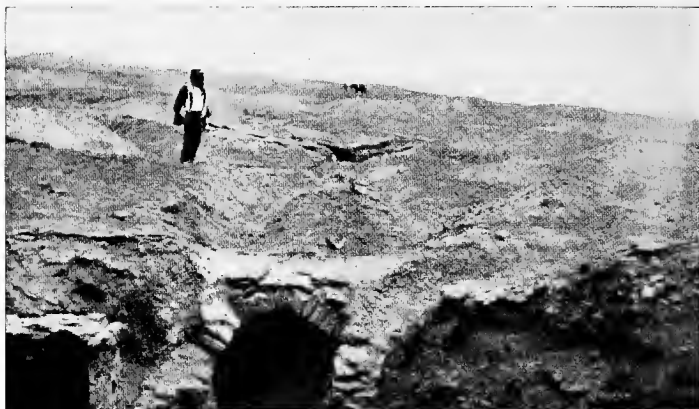
An Arched Sewer of Plano-Convex Bricks.
