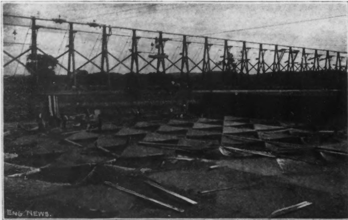
FIG. 5.—CONSTRUCTING THE INVERTED ARCHES FOR THE FLOOR OF THE FILTER BEDS.
