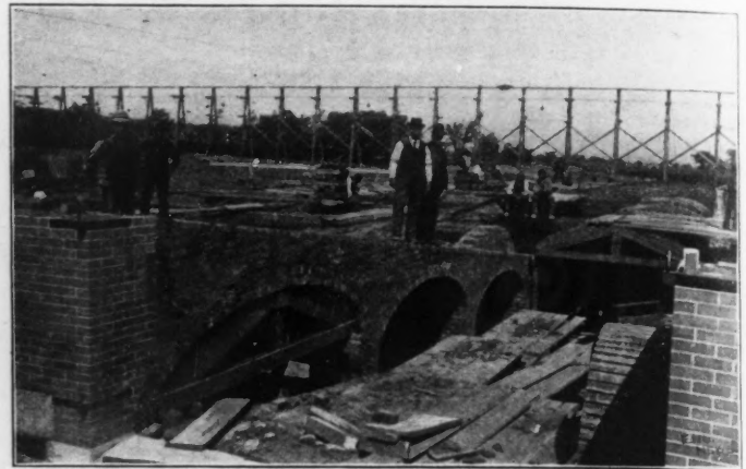
FIG. 6.—INCLINED ENTRANCE TO FILTER BEDS.
