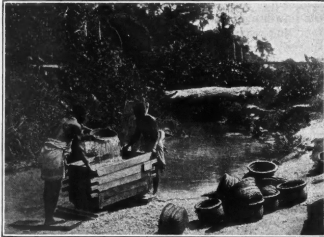
ROCKING SCREENS ON DEVELOPMENT WORK, KASAI DIAMOND FIELD
