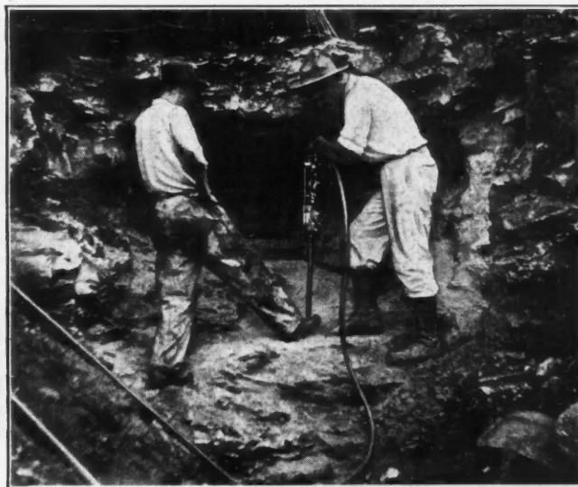
STARTING A NEW TUNNEL ON A SMITHSONITE OUTCROP ON RUSH CREEK
