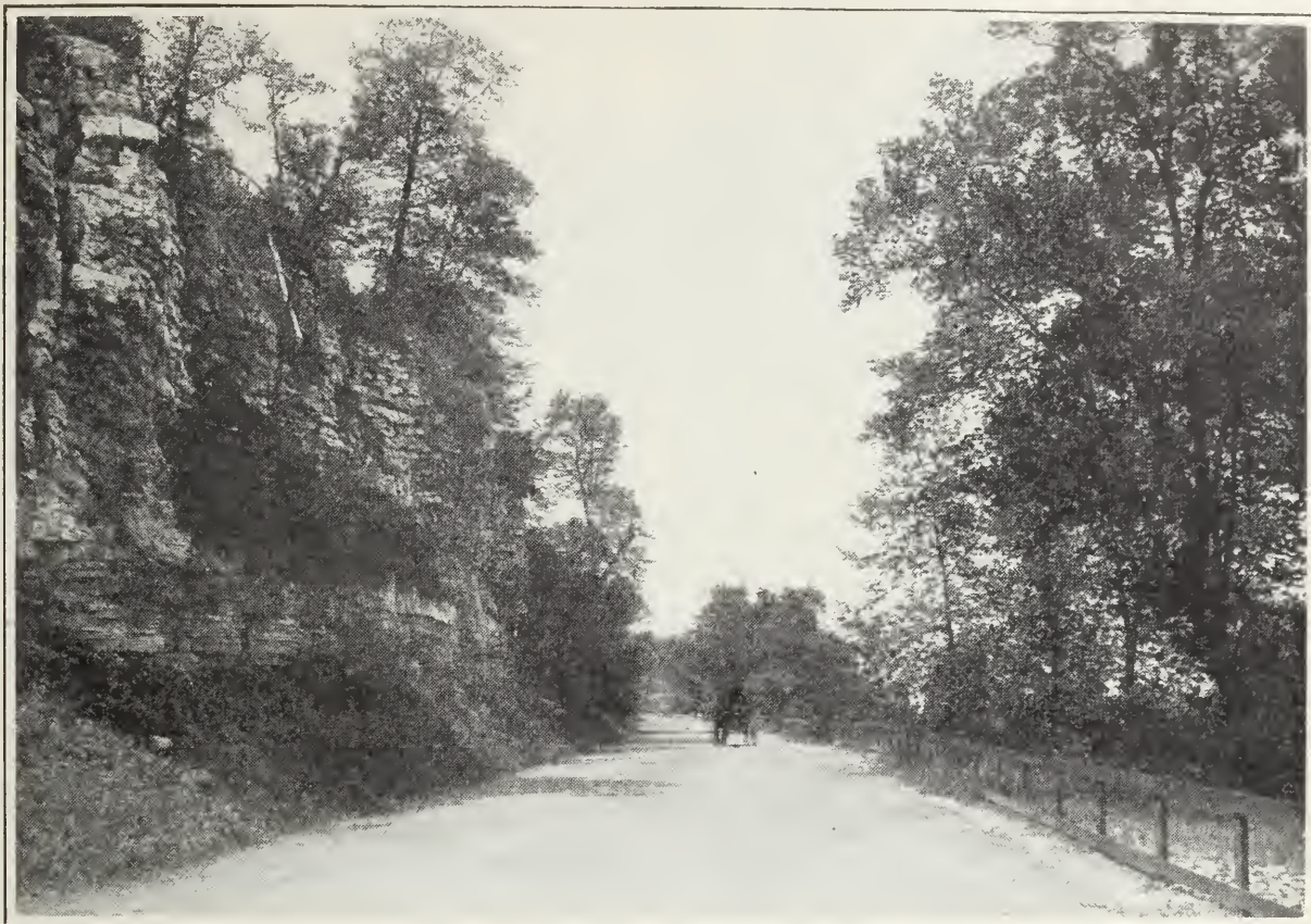
THE CLIFF DRIVE, NEAR KANSAS CITY, AFTER COMPLETION
