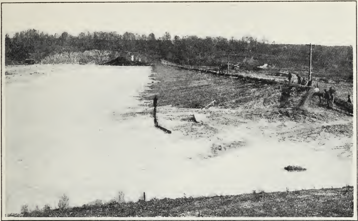
AN HYDRAULIC-FILL DAM UNDER CONSTRUCTION
