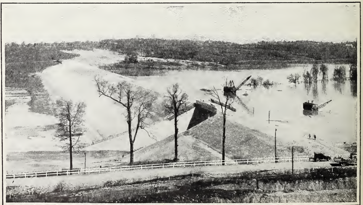
THE HUFFMAN DAM HOLDING BACK A SMALL FLOOD
