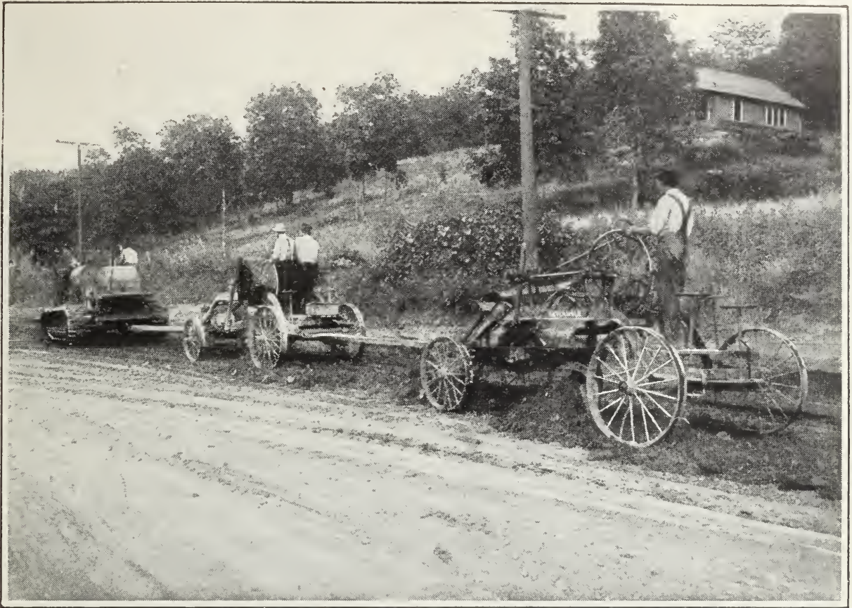
GRADING THE "CATERPILLAR TRAIL" NEAR PEORIA, ILLINOIS
