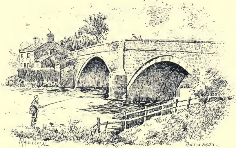
BOLTON BRIDGE AND FERRY HOUSE.
