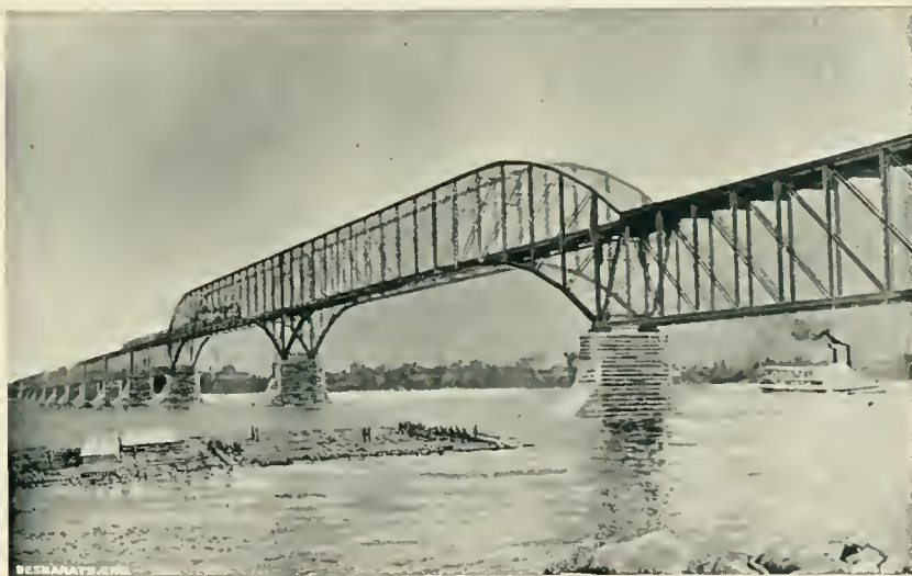
ST. LAWRENCE BRIDGE, C. P. R., LACHINE.
