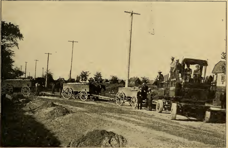
An American four-wheel driven gasoline truck, drawing thirteen tons in trailers.
