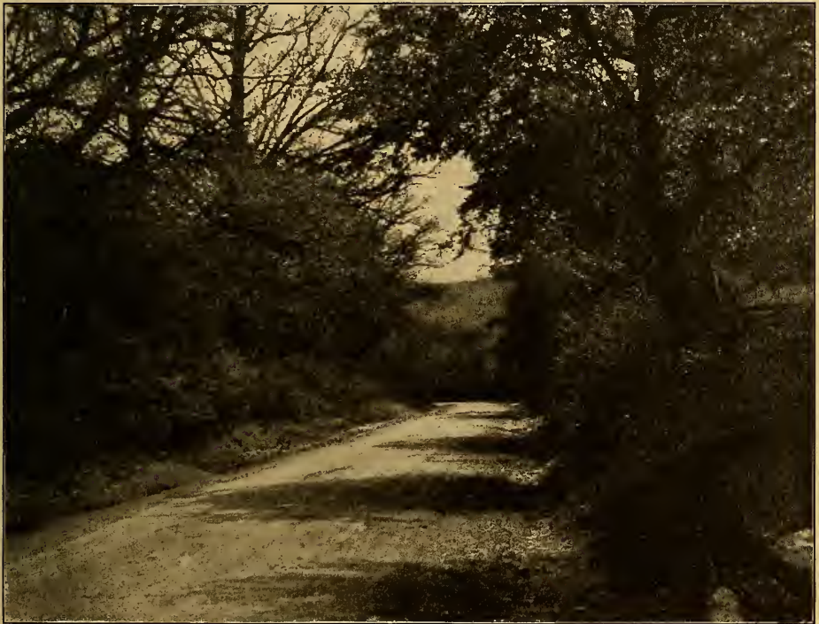
In Crawford County, Pa., after the State Highway Department has been at work.
