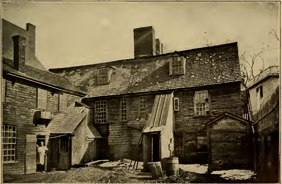
Rear View of the "witch" house.
