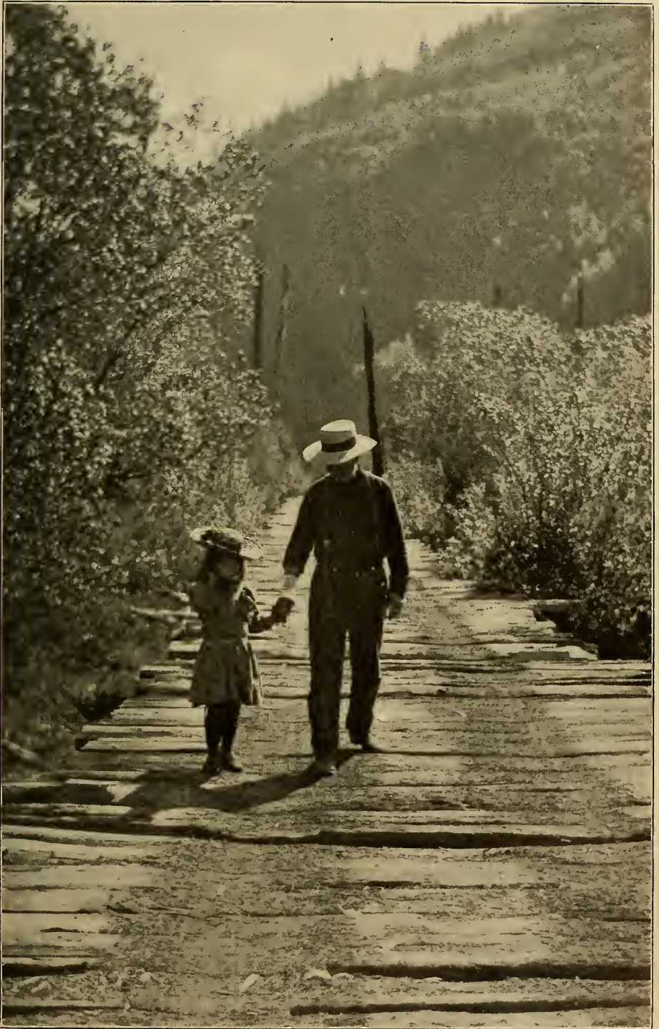
The corduroy is employed to bridge the marsh.
