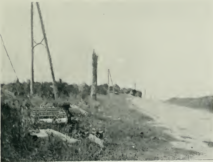
Ruins of St. Rohart Factory, looking West.
