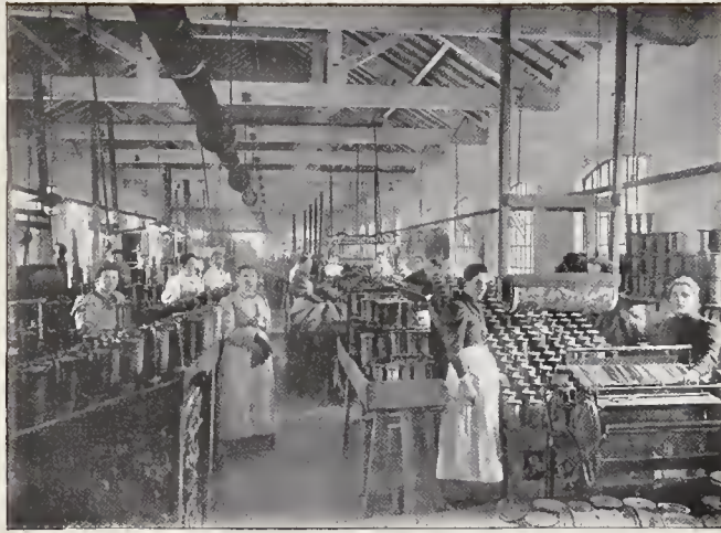
THE READING-IN ROOM. FIRST PROCESS IN MANUFACTURE OF AXMINSTER CARPET. NO. 1.
