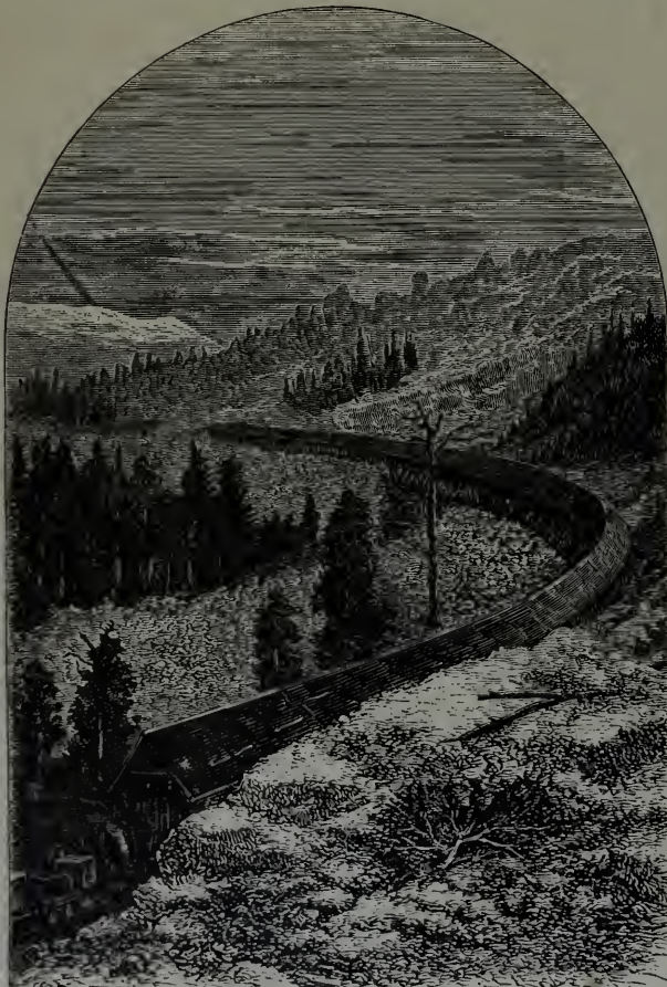
SNOW SHEDS ACROSS THE SIERRAS.
