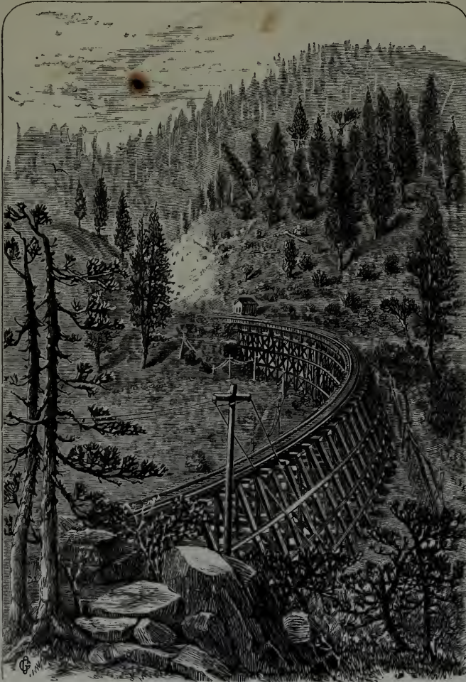
SECRET TOWN, TRESTLE-WORK.
