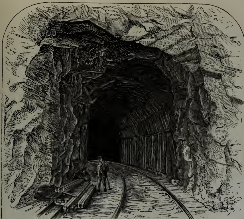
TUNNEL NO. 12, STRONG'S CANON.
