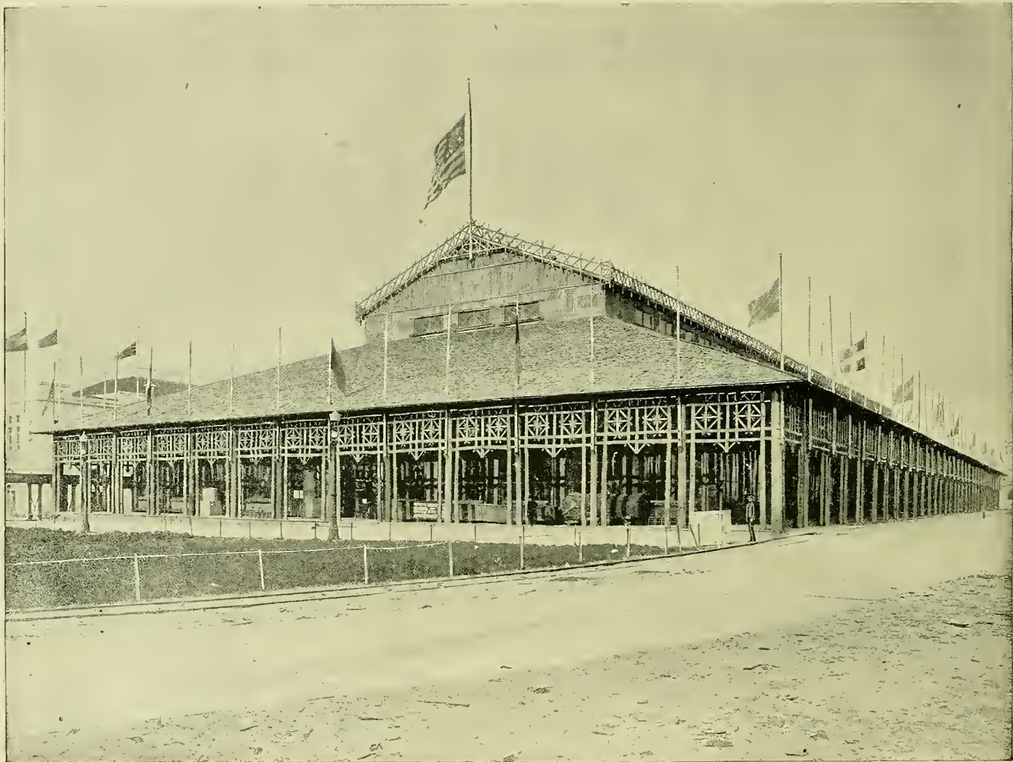
THE FORESTRY BUILDING, situated on the lake front near the extreme southern limit of the grounds, is in itself a great display of forest products, being built entirely of rough logs pegged together with wooden pins, not a single nail or piece of metal being used in its construction. It is surrounded on all sides by a roofed colonnade, the pillars consisting of three tree-trunks bound together and clothed in their natural bark. Various States of the Union and foreign nations contributed the material to construct this interesting building. The roof is thatched with many varieties of barks. This unique structure was designed by Mr. C. B. Atwood, is in size 528 x 208 feet, and cost about $100,000.
