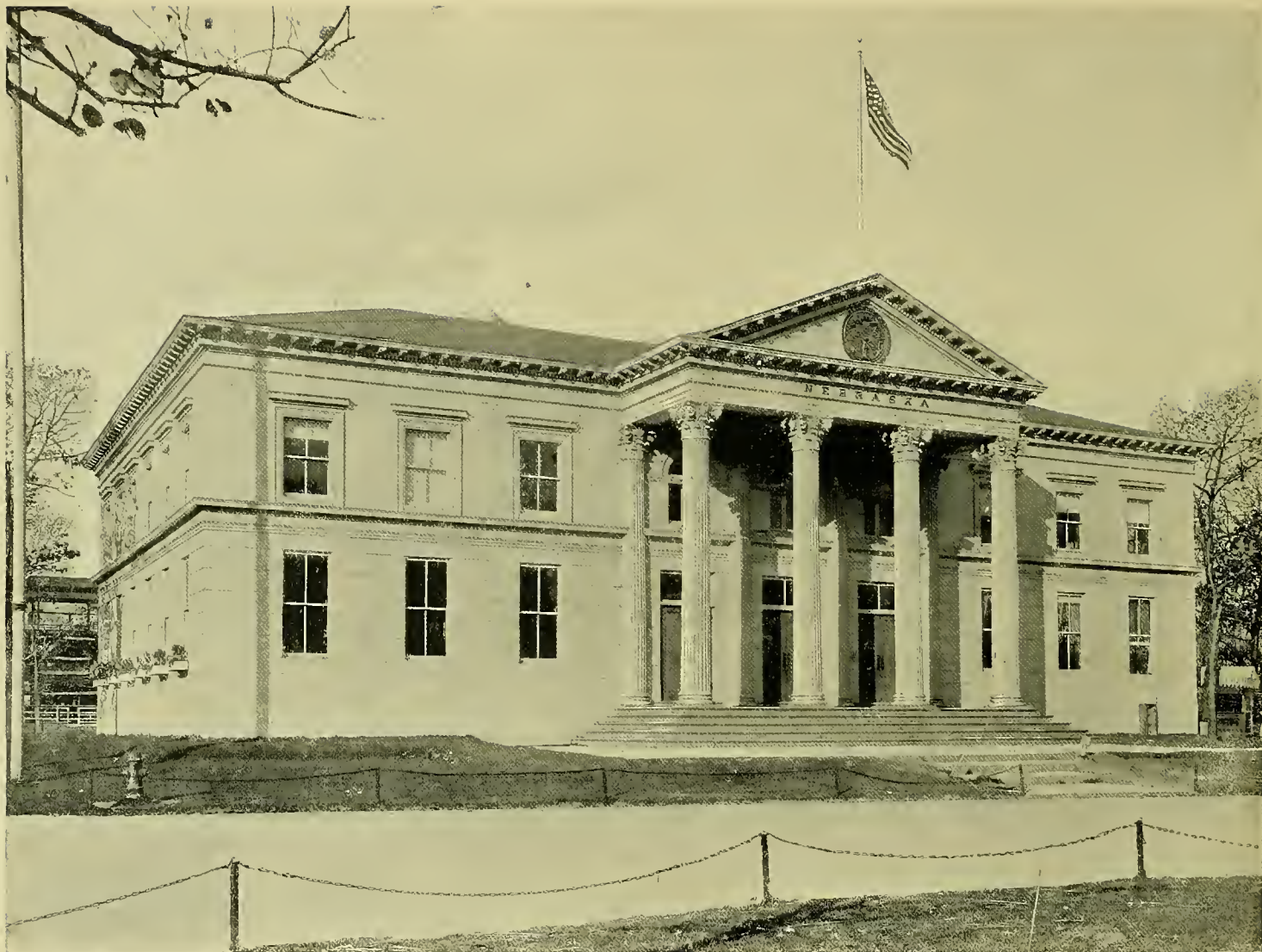
THE NEBRASKA STATE BUILDING is of the colonial style of architecture, and classic in its simple impressiveness. On each side of the building is a large portico with eight massive columns upholding the pediment, which bears the State coat-of-arms in bas-relief. The house measures 100 x 60 feet, and is constructed of staff treated to represent stone. On the first floor is a large hall for exhibition purposes, besides reception-rooms and toilet-rooms. On the second floor are other rooms for the display of native products, and ladies' reception-rooms, etc. The architect was Mr. Henry Voss, and the building cost $15,000.
