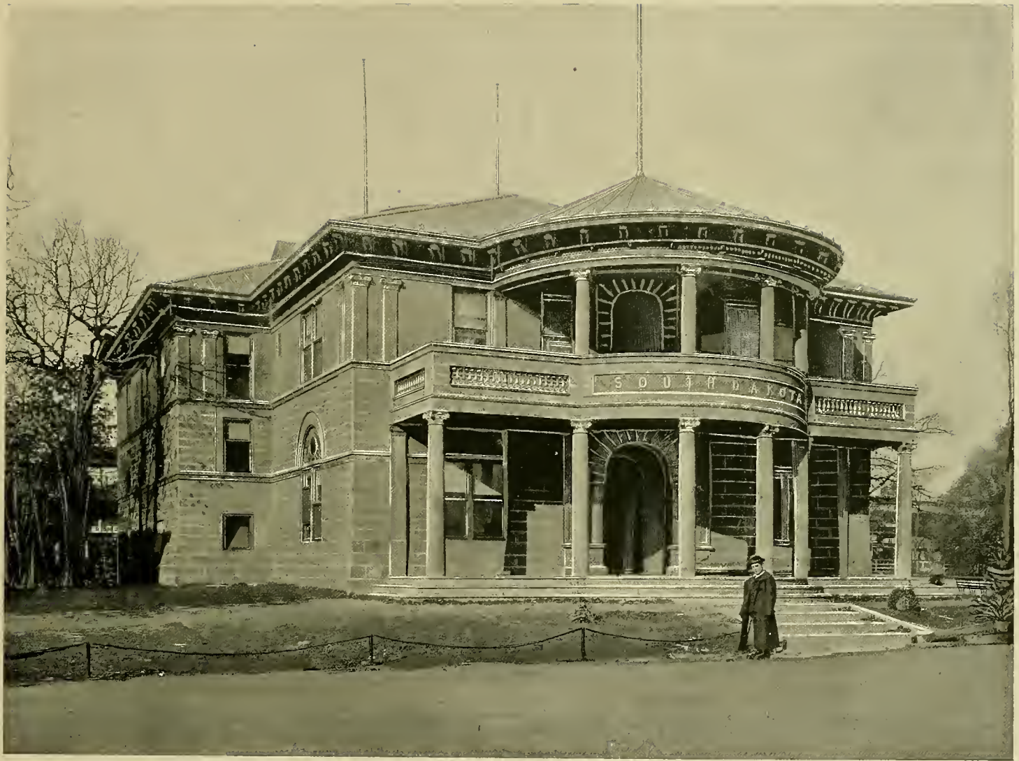
THE SOUTH DAKOTA BUILDING is entirely the creation of the muscle, brain, material, and money of that State. The exterior is coated with Yankton cement, the timber is the product of her forests, and the roofing the product of her mines. Within its walls a wonderfully varied exhibit of the natural resources of the State are exhibited, including all the fruits of the temperate zone, and almost all known metals. The building measures 100 x 60 feet, is Romanesque in style, and cost $25,000.
