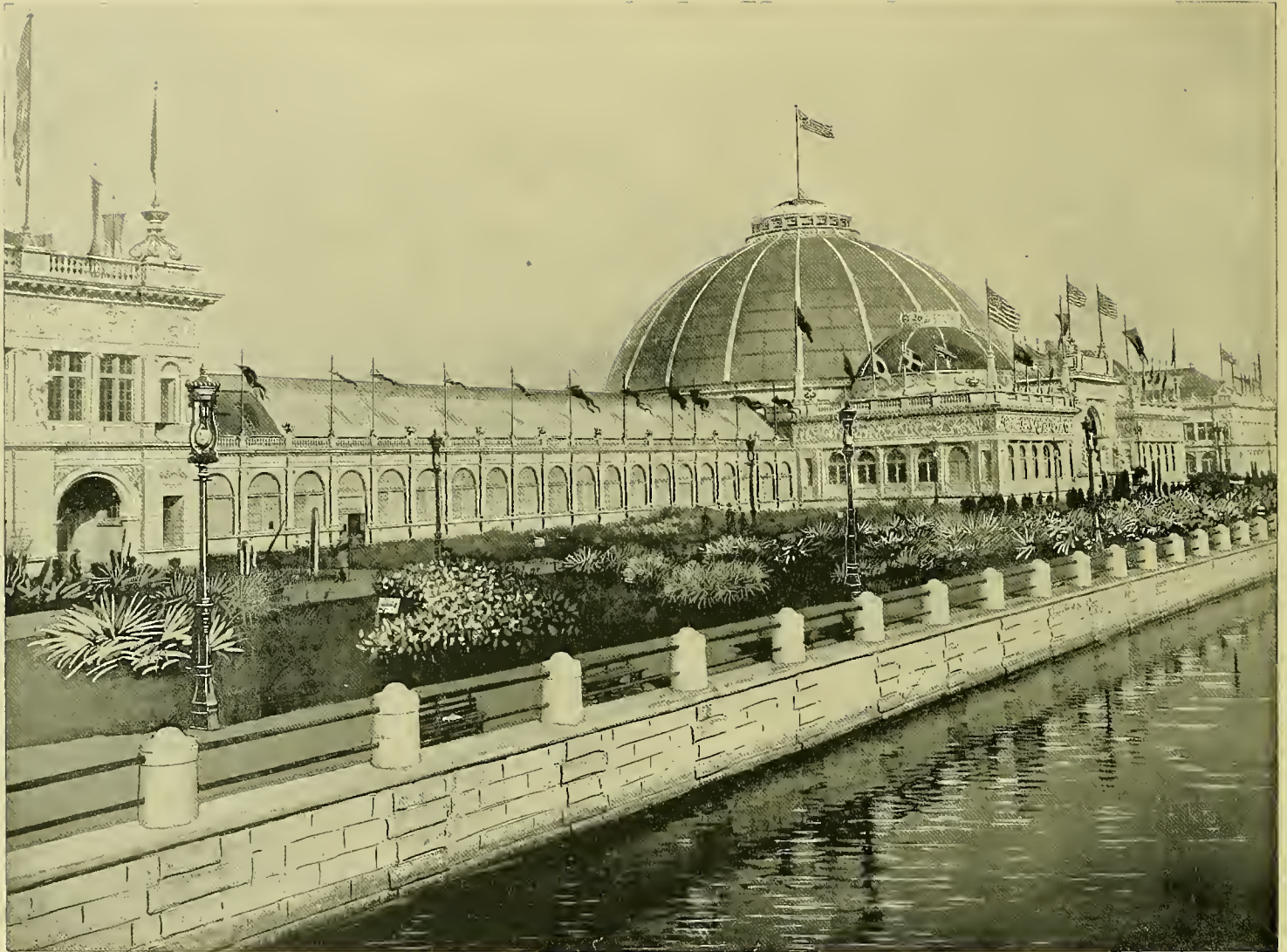
HORTICULTURAL BUILDING, eastern exposure, facing the Lagoon and Wooded Island. The architects, Messrs. W. L. B. Jenney and W. B. Mundie, designed not only a work of art but a building so perfectly suited to its purposes that it will serve as a pattern for all time to come. In size it is 1,000 x 240 feet. In the center rises a glass dome 180 feet in diameter and 114 feet in height, which accommodates the great palms, tree ferns, bamboos, and other growths of tropical lands. Statues, singly and in groups, symbolical of the seasons and of fruits and flowers, besides many minor single figures, add greatly to the charm of this beautiful building.
