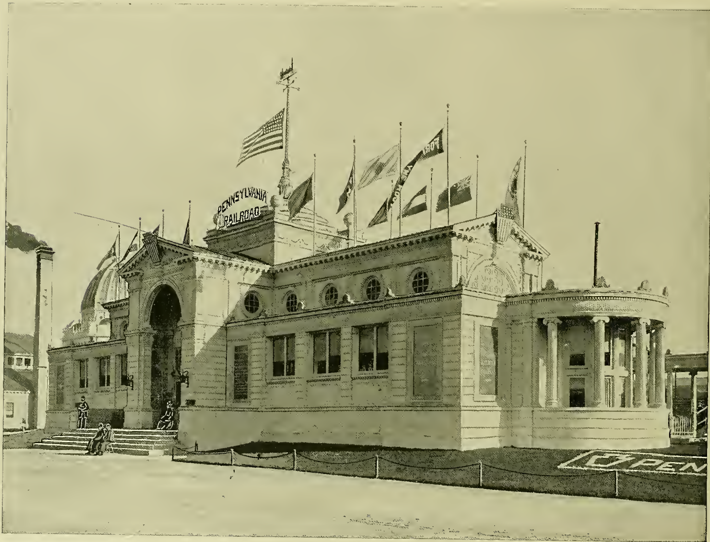
THE PENNSYLVANIA RAILROAD PAVILION was one of several erected by corporations and firms for the exclusive exhibit of objects pertaining to their business. In this building, among other things, the Pennsylvania Railroad Company displayed a striking series of views which formed almost a complete panorama of the scenery along their line of road. A corps of officials were in attendance to give information upon all of the innumerable subjects connected with this vast system. The surrounding lawns were beautifully kept and made brilliant with flowers, and the comfortable seats and cool interior made a refreshing resting-place for tired sight-seers.
