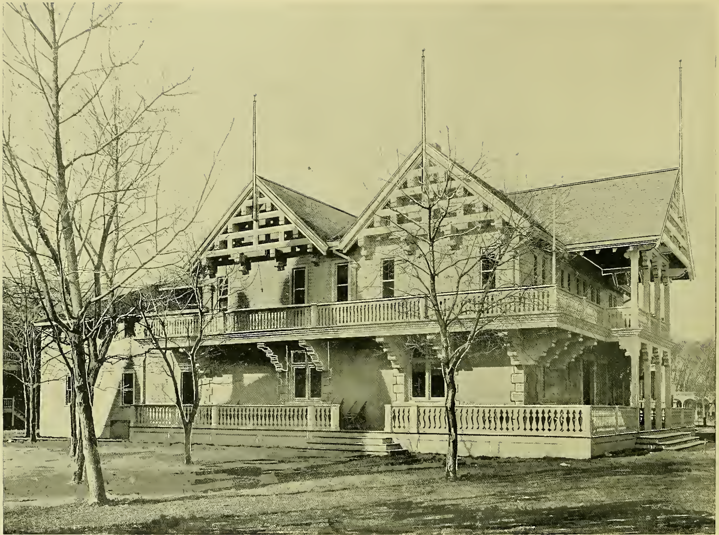
THE NEW HAMPSHIRE BUILDING is constructed in imitation of the heavily-bracketed and balconied chalets of Switzerland, symbolizing the Switzerland of America, as New Hampshire is often called. It occupies one of the most favorable locations on the grounds, facing Lake Michigan. The first story is built of plaster, with quoins to the doors and windows of various kinds of New Hampshire granite. The building is rectangular in form, the center being occupied by a hall 22 x 25 feet, which extends up through two stories to the roof. The building cost about $12,000, and was designed by Mr. G. B. Howe of Boston and Omaha.
