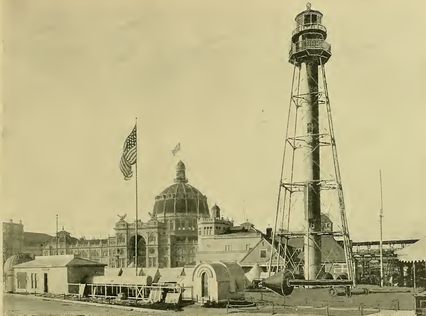
THE UNITED STATES SIGNAL SERVICE EXHIBIT and Life Saving Station proved of great interest to visitors of the World's Fair. The light-house is of the modern steel pattern, 100 feet high, and furnished with the most powerful revolving white and red lights. It will shortly be taken down and be removed to the mouth of the Columbia River. In the distance just beyond is the Life Saving Station, where daily drills of life-boat crews, etc., were held. To the left are the small buildings of the Naval Observatory, and over them, farther off, the Main United States Government Building.
