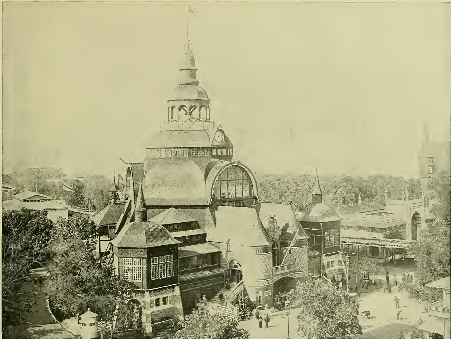
SWEDISH GOVERNMENT BUILDING. A picturesque, triangular edifice, located just north of the Fisheries Building, is the contribution of the Government of Sweden. It was modeled by Mr. Gustaf Wickman, of Stockholm, after a style prevalent in the sixteenth century, and was made in Sweden, where it was temporarily put together, and afterward sent to this country in pieces. The lower part of the front wall is composed of brick, terra cotta, and cement of Swedish importation, and the rest of the structure is of wood, covered with shingles. The huge crown on the top of the steeple, as well as the frame-work around the bell, are gilded, and touches of color here and there lend a pleasing effect to the eye.
