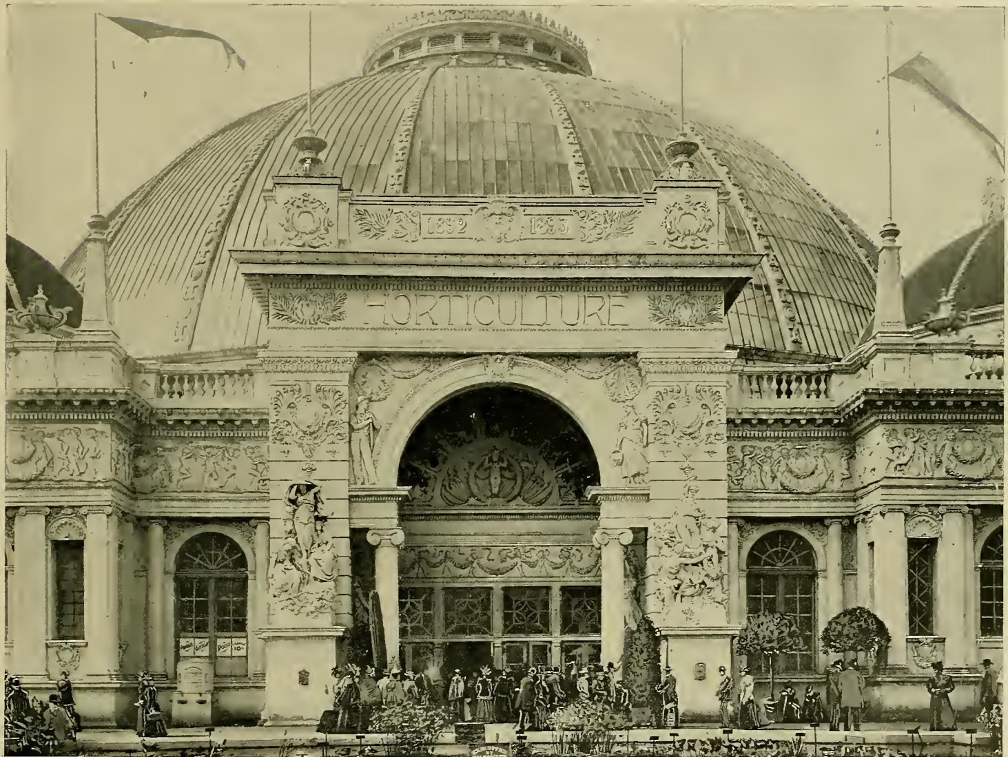
MAIN ENTRANCE TO THE HORTICULTURAL BUILDING. The glazed dome and central entrance to the Horticultural Building are here displayed in a manner to bring out the wealth of ornamentation in all its beauty and profusion. The dome is 180 feet in diameter and 114 feet high. In front of the pavilion, which is covered by this immense area of glass, is a highly ornamented pylon, with a recessed vestibule decorated with statuary. On the face of the pylon are groups, one on either side, representing the "Awakening," and the "Sleep of Flowers." Inside the vestibule are heroic statues of "Flora" and "Pomona."
