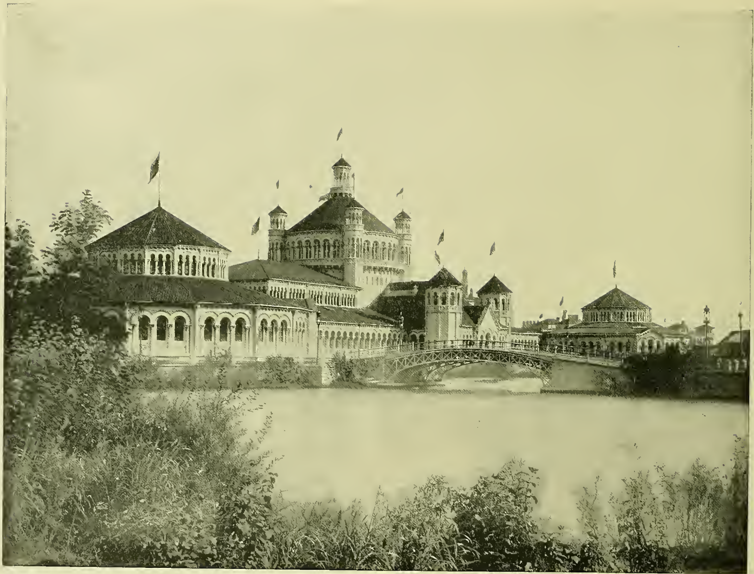
FISHERIES BUILDING, as seen from the Wooded Island, looking northeast across the Lagoon. This building differs essentially in spirit from any of the other main buildings on the grounds, and forms a striking and pleasing contrast thereto. The architect, Mr. Henry Ives Cobb, designed a most ingenious structure, no less remarkable for its grace and beauty of detail than for its fitness to the purpose for which it was erected. The wealth of ornamental detail is all formed of representations of fish and other marine animals, which give a key to the nature of the exhibits within. The circular outlying pavilions, the eastern one containing the aquariums, are connected with the main body by arcades, which form delightfully cool and shady resting-places. The style of architecture is Spanish renaissance. The extreme length is 1,100 feet and the greatest width 200 feet. Its cost was $200,000.
