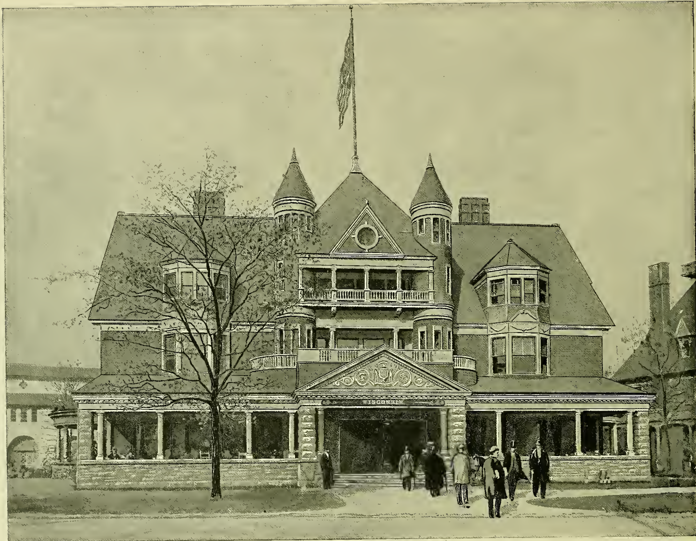
WISCONSIN BUILDING. In striking contrast to other buildings in the northern part of the grounds is the modern structure of the State of Wisconsin, situated near the west bank of the North Pond. It has a frontage of ninety feet, exclusive of the porches, and a depth of fifty feet. The walls of the lower story are of Lake Superior brownstone and Menominee red pressed brick, and above that the exterior finish is chiefly in native dimension shingles. Massive brownstone pillars and polished granite columns support the front and rear porches. In the angles of the gables is seen the coat-of-arms of the State, modeled by Miss Eunice Winterbotham, of Eau Claire. A pleasing effect is produced by the harmoniously contrasting colors in which the exterior is painted. Its cost was $70,000.
