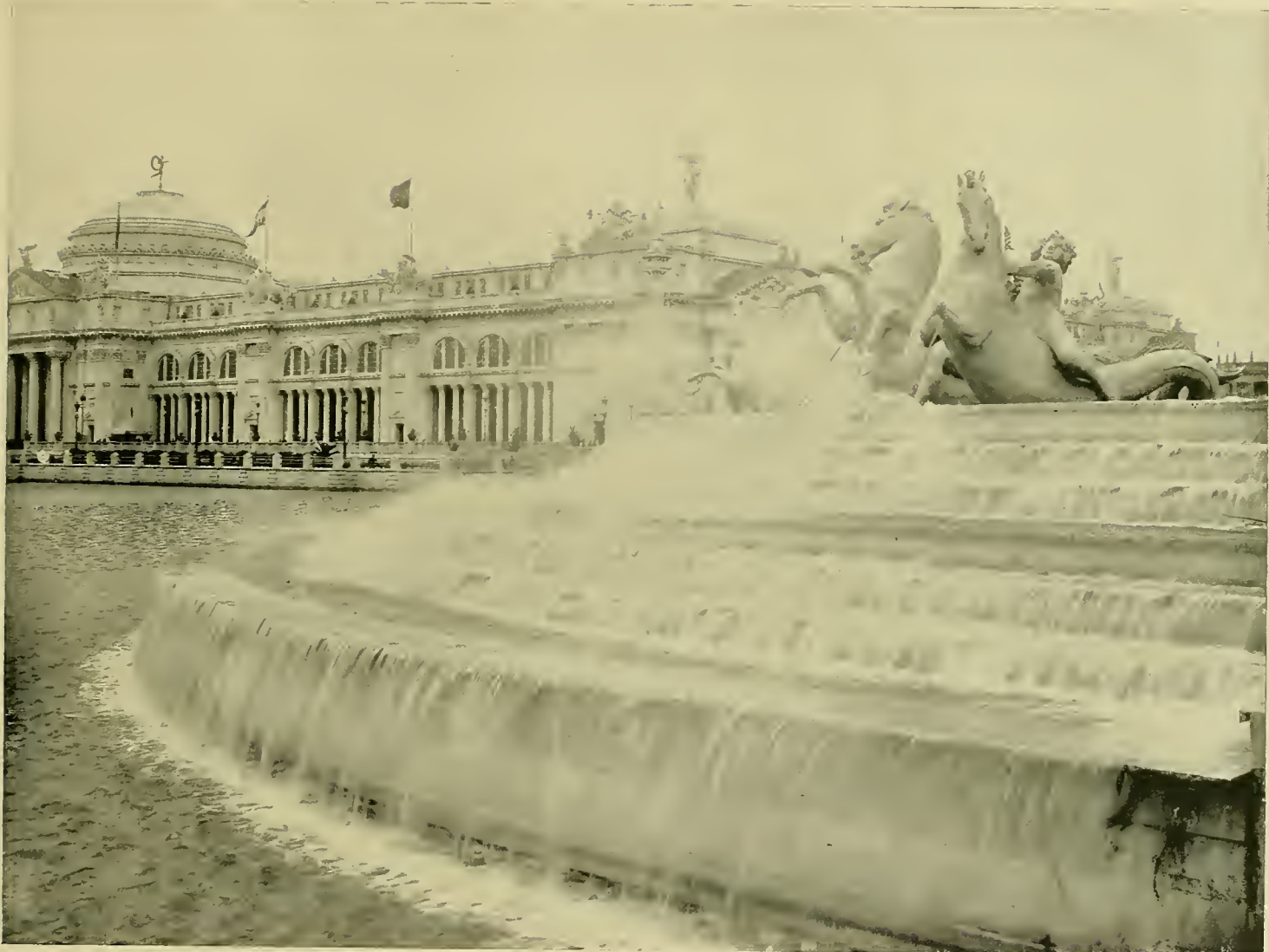
THE BASIN OF THE MacMONNIES FOUNTAIN—150 feet in diameter—was raised twelve feet above the level of the surrounding Main Basin. Over the edge of it water rushed in a series of miniature cascades. Sea-horses, mounted by figures representing modern advance, plunging forward, lead the way for the barge bearing Columbia. The detail of that part of the Basin facing the northeast is well shown in the accompanying illustration. In the distance the western half of the north façade of the noble Agricultural Building—the airy form of Diana clearly silhouetted against the sky—adds a charming completeness to the picture.
