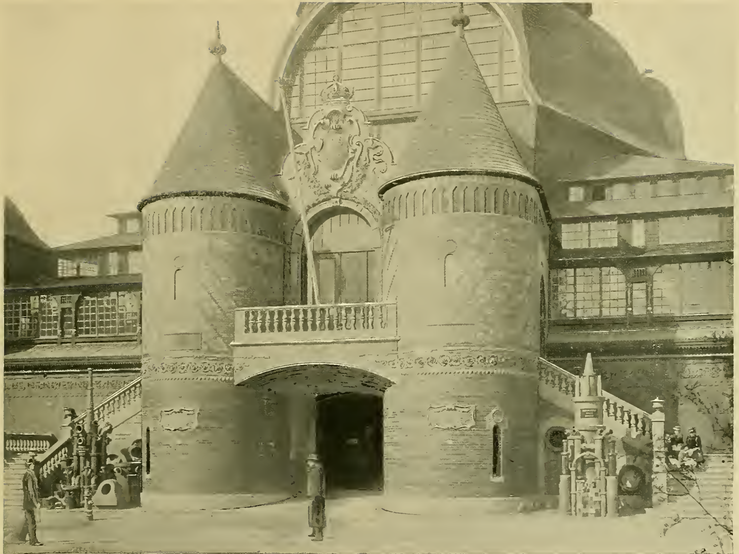
THE ENTRANCE TO THE SWEDISH BUILDING presents an interesting study of the architecture of Sweden during the sixteenth and seventeenth centuries, which it closely follows. The building, the design of Mr. Gustaf Wickman of Stockholm, was constructed in that country, and then taken apart and brought over here to be reconstructed in Jackson Park. The entrance is of brick and decorated with terra cotta, the product of famous Swedish manufactories, and is of itself no insignificant exhibit. The building is in the form of a triangle. The entrance leads into an immense hexangular hall, from which open rooms used for the display of exhibits.
