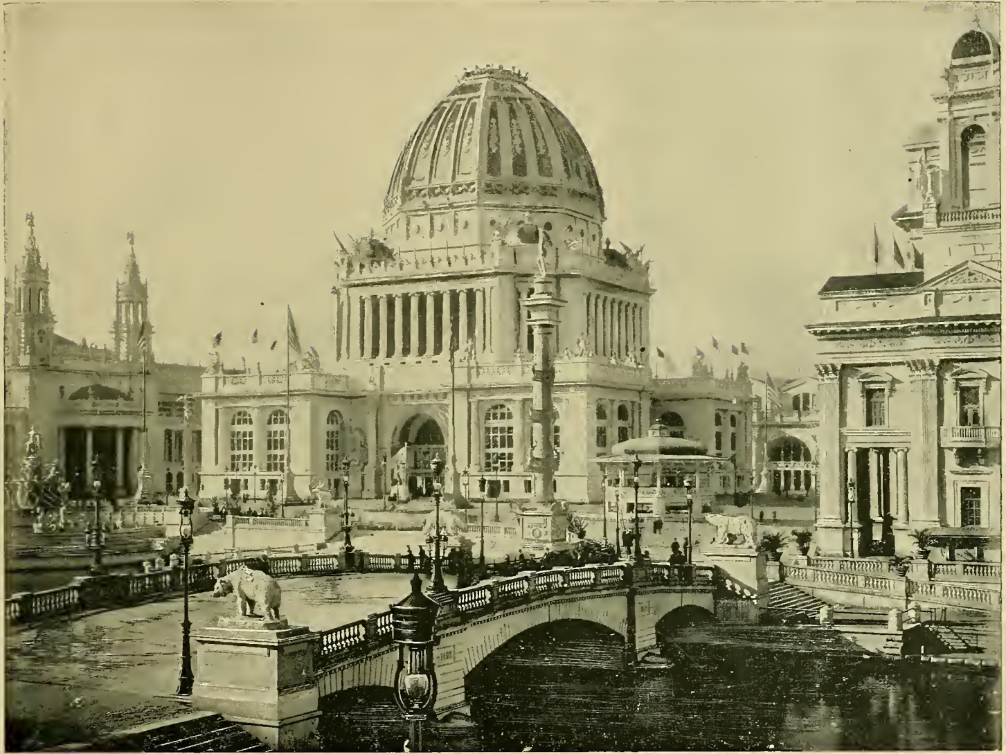
ADMINISTRATION BUILDING, eastern exposure. Situated at the west end of the Great Court. Designed by Richard M. Hunt. It is, in its main body, an octagon, about 100 feet across, with a pavilion 84 feet square at each corner. It rises to a height of 275 feet, and its gilded dome is a striking landmark from all parts of the grounds. It is adorned with twenty-eight groups of statuary and many single figures and bas-reliefs. The beauty of this building has been recognized as fully abroad as in this country, and its distinguished architect has been the recipient of many honors from foreign art associations. Cost, $450,000.
