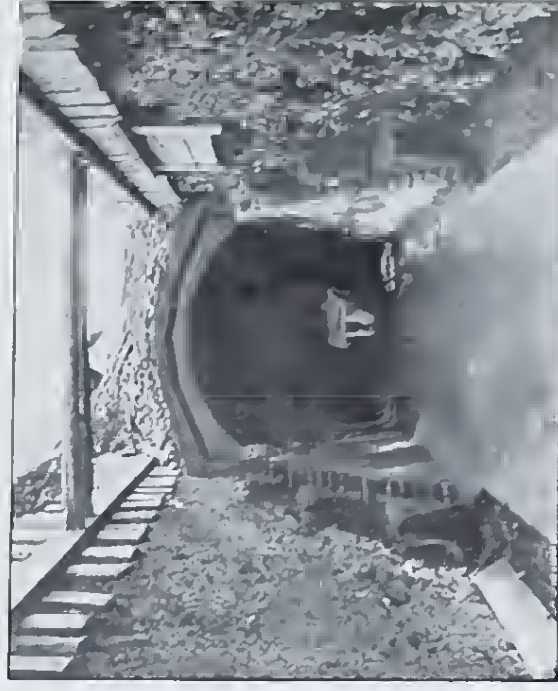
Specimen of Cut and Cover, Feb. 1898.
