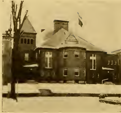
From a photograph Kindness F. E. Wing, Esq. HIGH SCHOOL BUILDING, ATHOL, MASSACHUSETTS,
