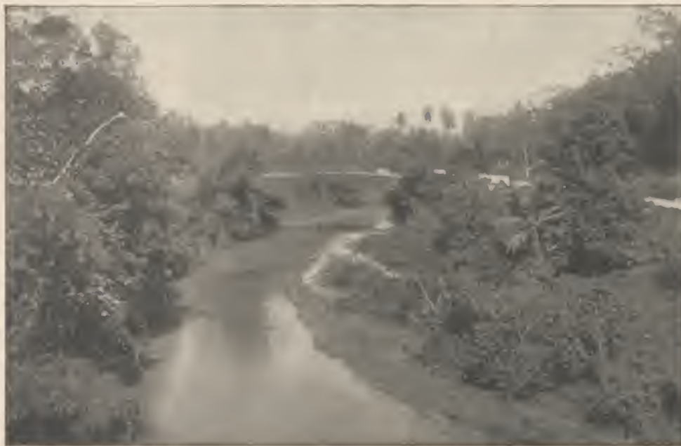
BRIDGE ON RIO COBRE RIVER.
