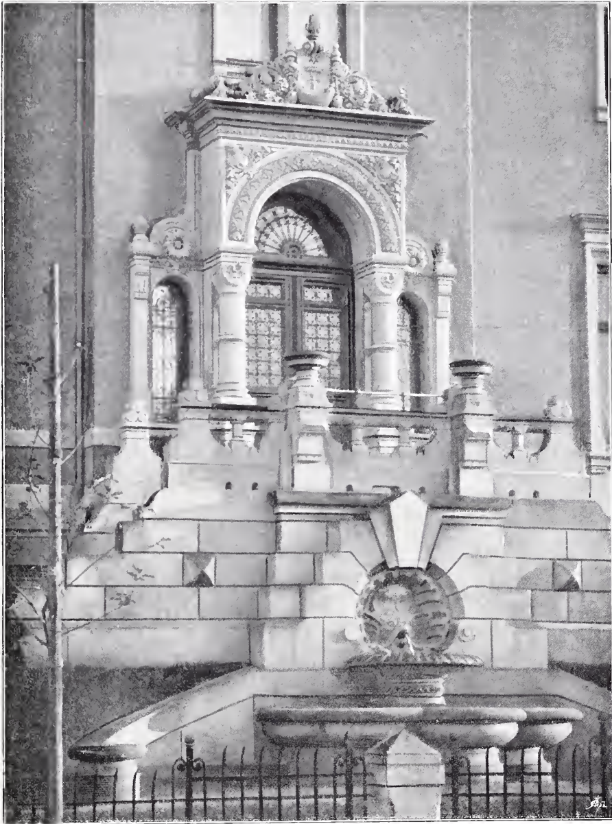
Detail, Principal Entrance, Villa Schmid, Dresden, RICHARD MICHEL, Architect, Höxter.
