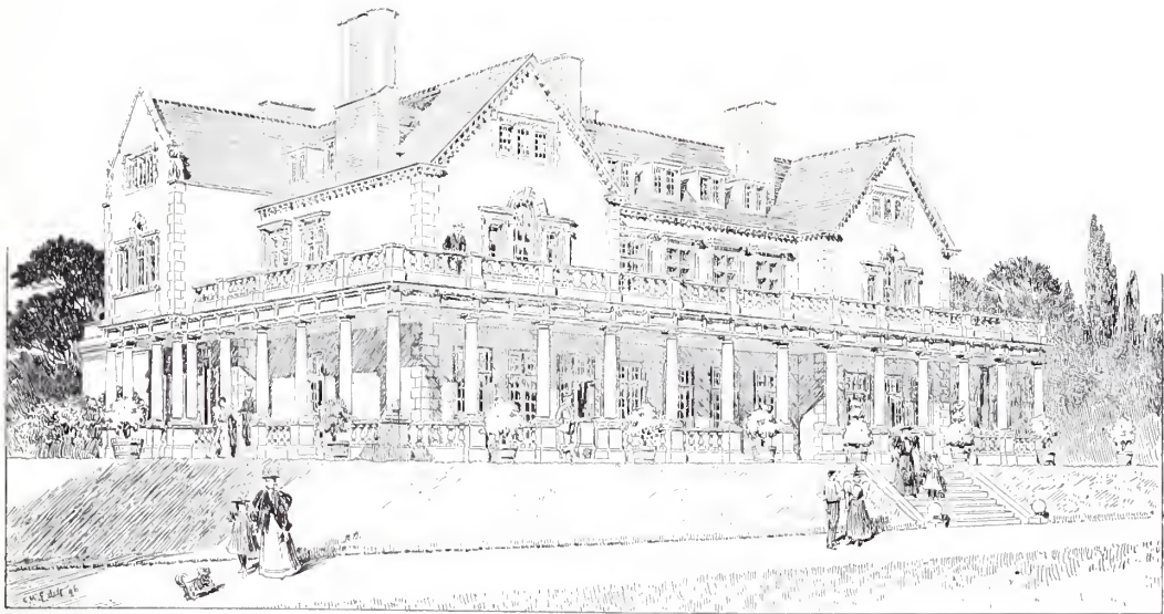
1693. An Hotel in the Isle of Wight , FRANK S. TAYLOR, A.R.I.B.A., c Architect.
