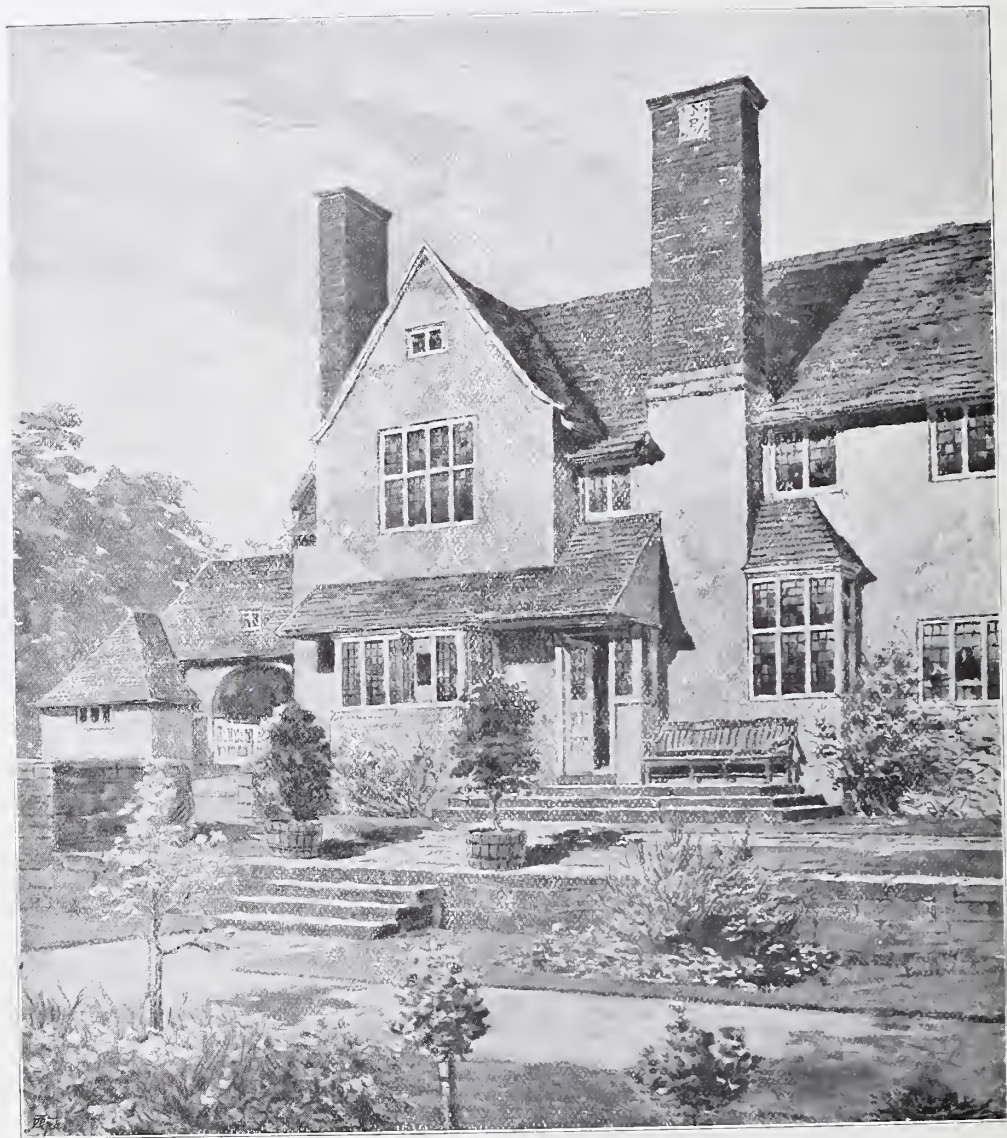
1644. Corner of House, Edgbaston, Birmingham, BATEMAN AND BATEMAN, Architects. (For Plans, see p. 45.)
