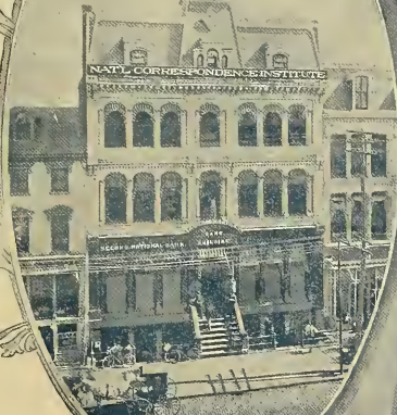
View from Post Office Department.
