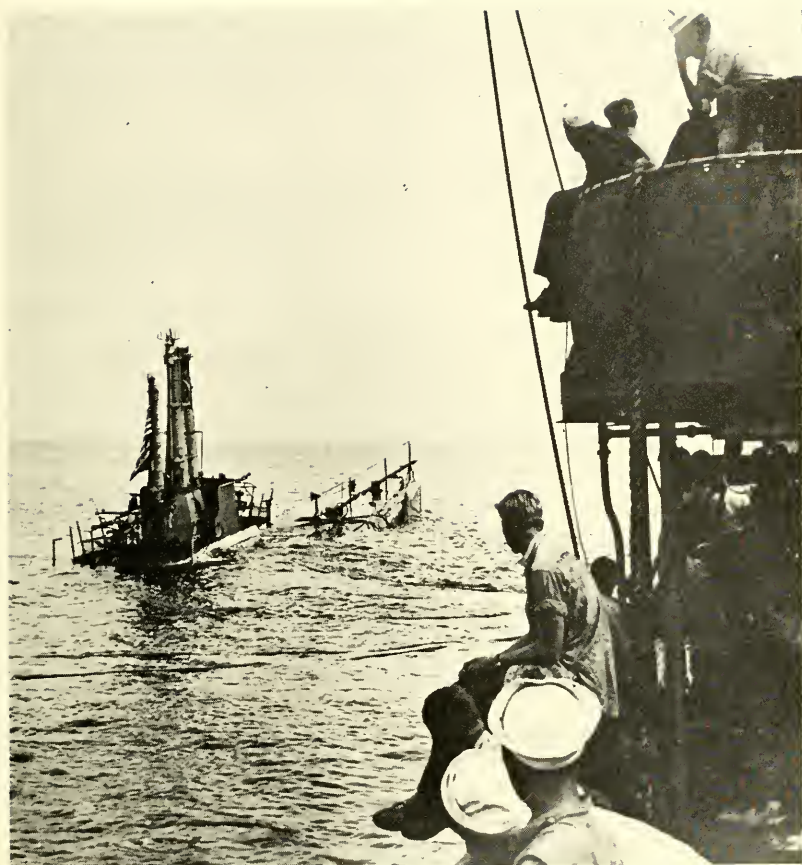
Crew of the submarine rescue vessel WIDGEON watch the test submerging of the submarine APOGON. The submerging operation was difficult; never before had there been occasion to submerge a submarine without crew aboard. The method used was to fill part of the ballast tanks with water, then suspend heavy weights from the bow and stern by cables of carefully chosen length. These weights overcame the submarine's residual buoyancy and drew her down to the desired depth. She could be surfaced again by pumping air back into her ballast tanks.
