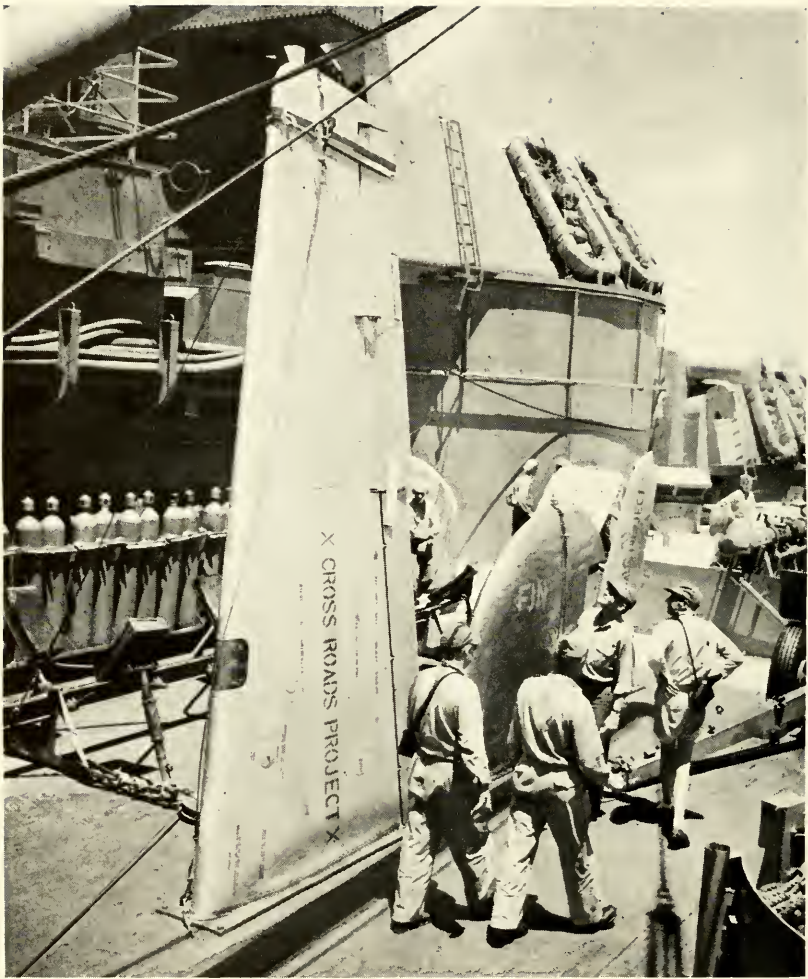
An experimental wing panel is mounted by the Army Ground Group on the deck of a target ship, to find the vulnerability of such panels to atomic bomb explosions. Visible along the deck are a tail fin, a stabilizer, and a range-finder. All items are clearly labeled for post-explosion identification.
