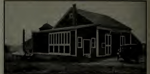
The combination barn, garage, and wormwood distillery on Mr. Young's farm
