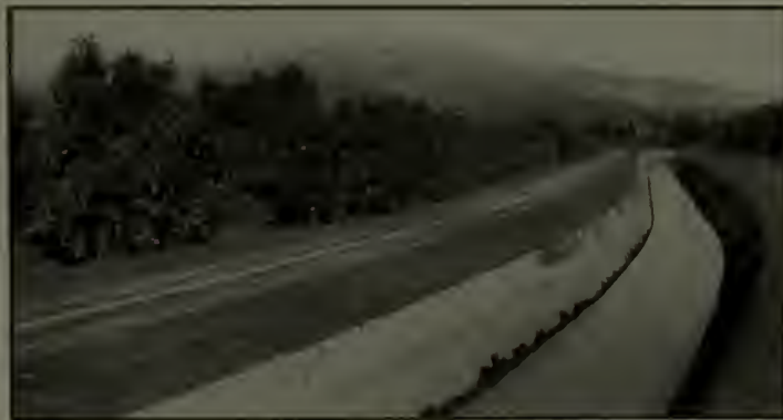
The irrigating canal which traverses the Riverside, Cal., orange groves
