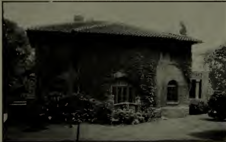
Before the concrete was quite hard the forms were removed and the surface scrubbed with water and stiff brushes, the lifeless color of the cement being thus eliminated and the variety and sparkle of the pre-selected aggregates revealed
