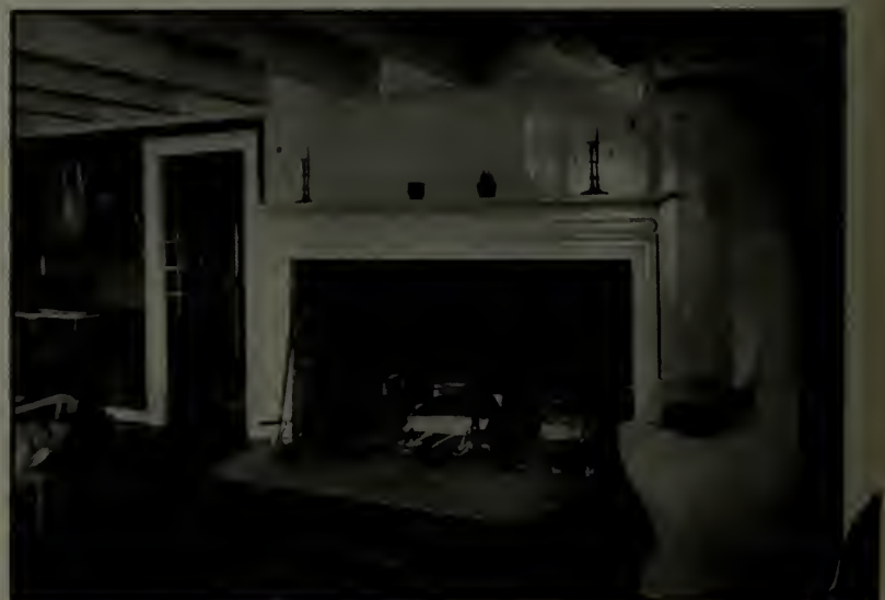
The fireplace in the living room. The only change here was the new paneled overmantel of plastic
