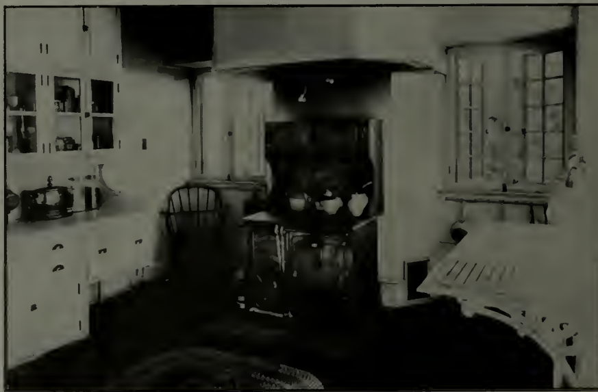
Showing the hood and ventilator, and the relation of the sink and dresser to the stove
