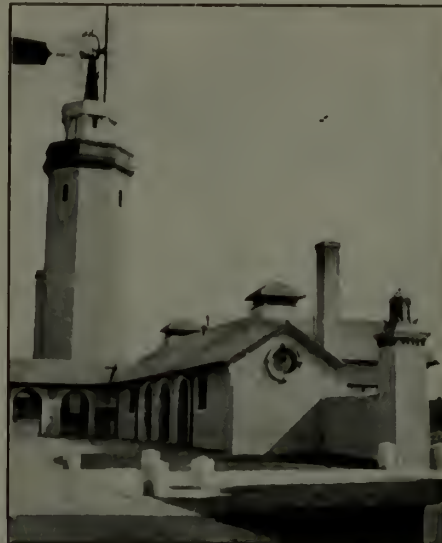
Mr. F. G. Bowne, Oakdale, L. I., has his water tower incorporated in the farm group and surmounts it with a windmill.
