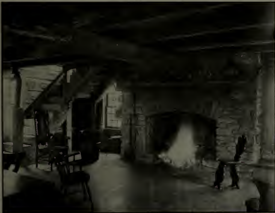
This fireplace in a log cabin on the estate of Robert W. Pomeroy, Esq., at Buffalo, N. Y., defies the rule which proscribes the inclusion of timbers in chimney construction
