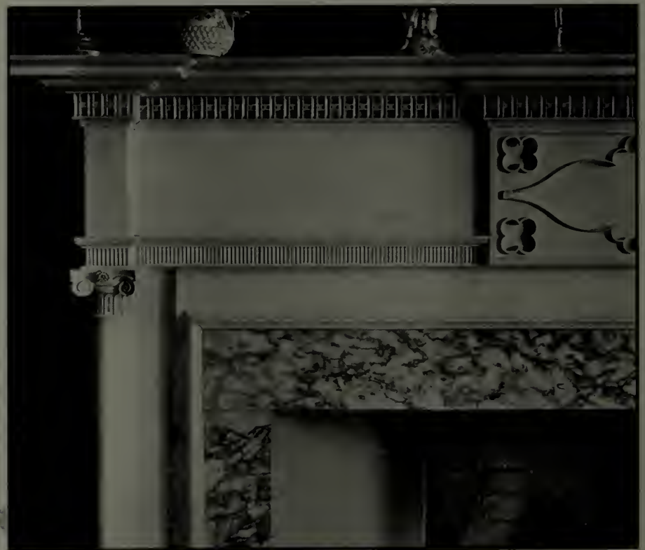
In the Larkin-Richter house at Portsmouth, N. H. The upper carved molding, here used instead of a dentil course, is a product of the New England craftsmen, probably inspired by the classic bead-and-reel
