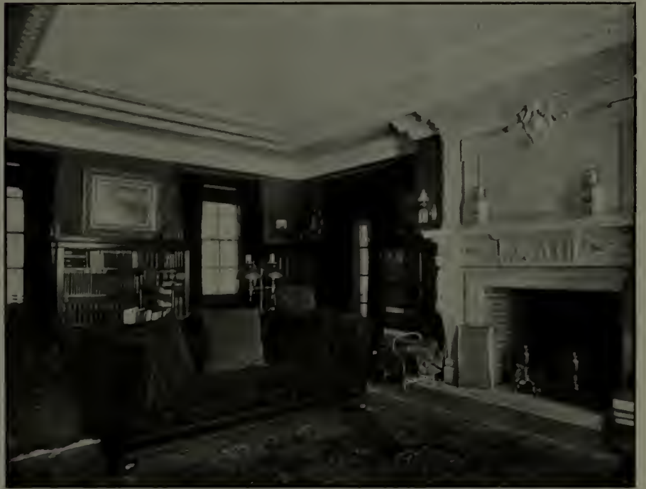
In the living room fireplace and cornice one feels again the same sturdy note of architectural embellishment.
