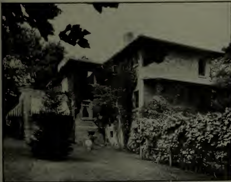
A mixture of one part each cement and three-quarter inch trap rock, and three parts limestone and white marble screenings the size of sand gave the scrubbed surface a pleasing texture and color
