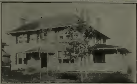
Walls finished with Cabot's Old Virginia White Roof with Cabot's moss-green Creosote Stain W. C. Northup, Architect, Winston-Salem, N. C.
