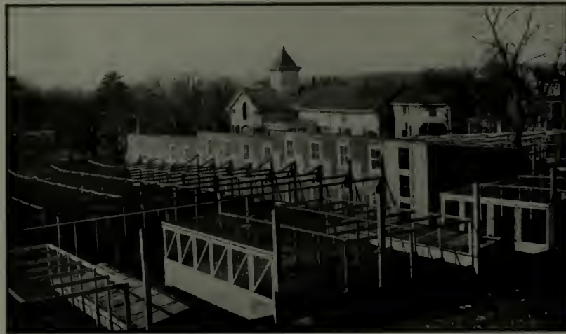
The front of Mr. Martling's 130-foot breeding house. There is an indirect ventilating system at the back, and the front windows are placed at different heights to facilitate control of ventilation and temperature
