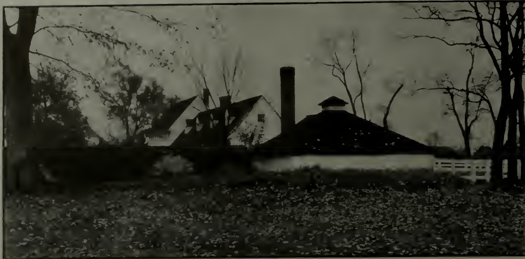
The brick ice house at the northeast corner of the group, showing the green-house in the background
