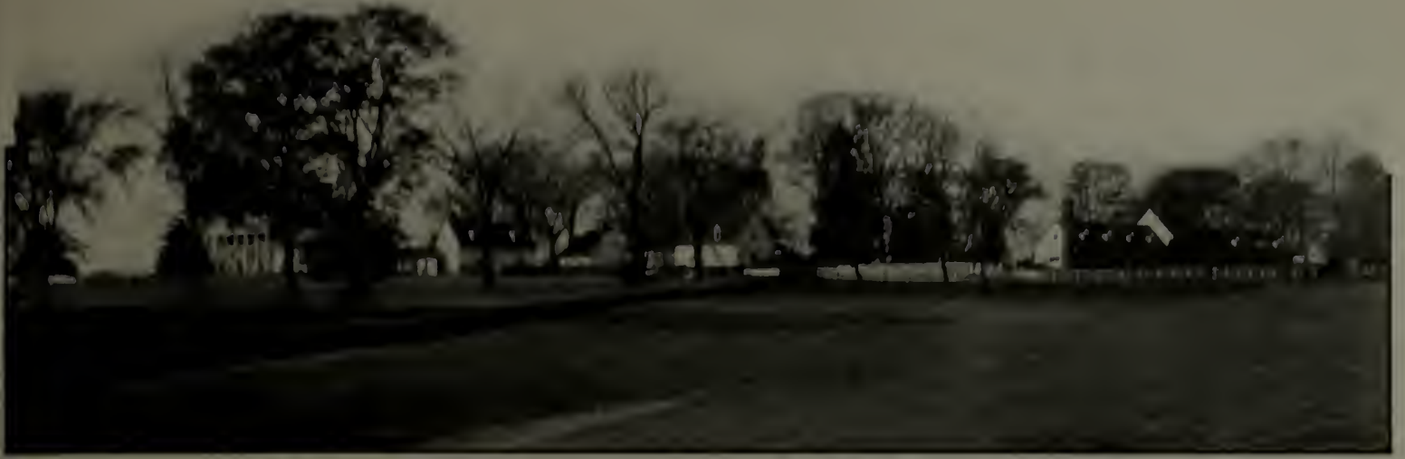
A view of the whole group of buildings that made up Mt. Vernon, taken from the slightly higher point of land to the northeast. From the lower left corner runs the ha-ha wall that kept the cattle in the meadow and off the lawn
