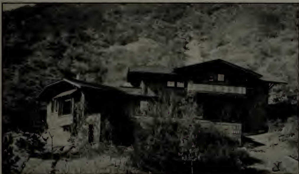
The Frost home, designed by A. R. Kelly. Although there is no planting around the house, it still ties into its surroundings in a satisfactory way
