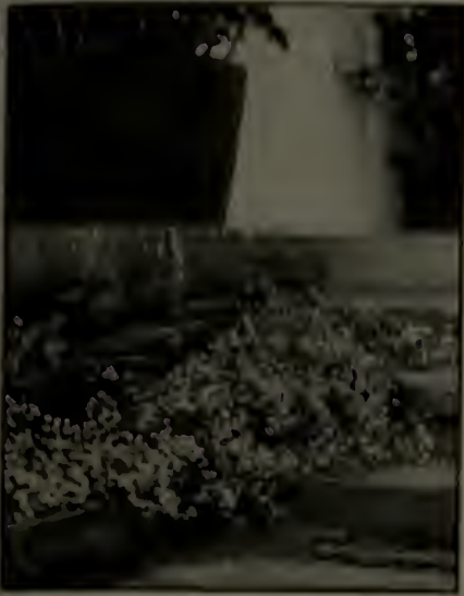
The rugged steps are of shale taken from the site and laid without cement
