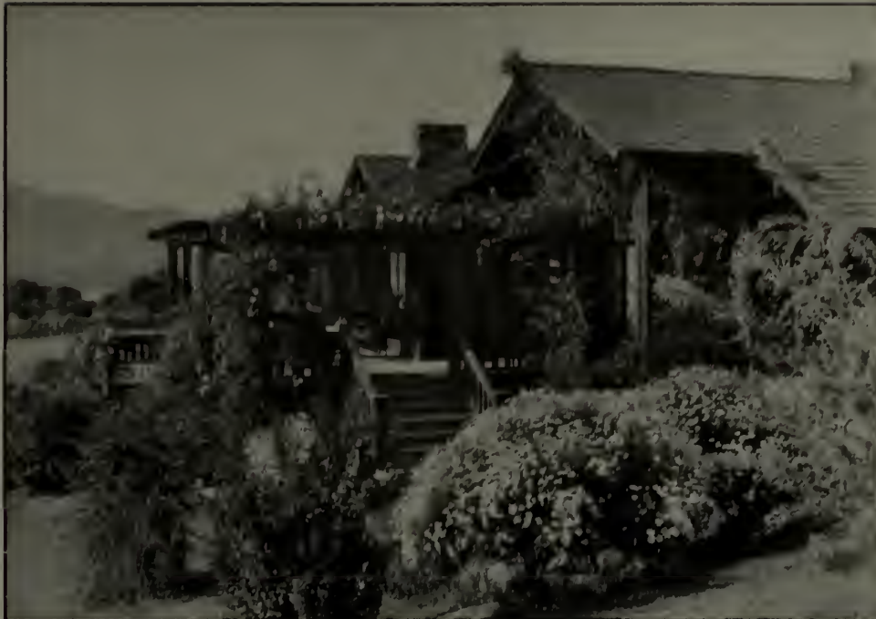
Here the house follows the hill contour, eliminating long flights of steps
