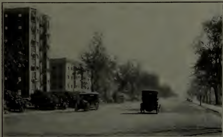
Kingshighway, St. Louis, Mo. Constructed with "Tarvia-X," penetration method, in 1915
