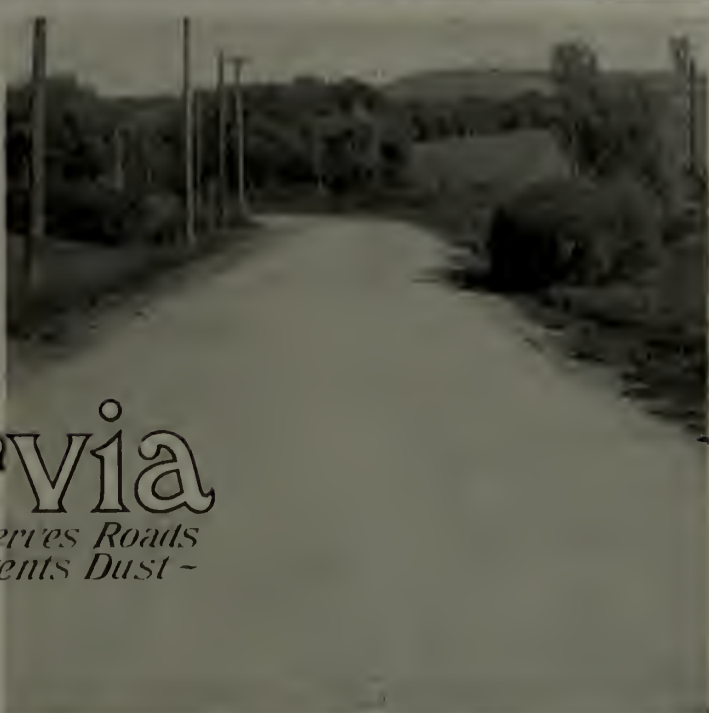
Forest Lawn Road, Florence, Neb., showing transformation of road surface after the use of "Tarvia-X" penetration method.
