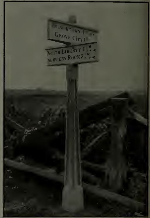
Concrete guide posts can be erected for about $15
