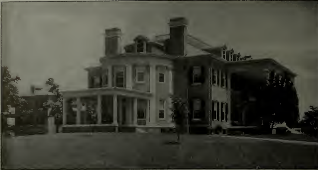
The west wing corresponds in form to the circular portico on the east, six flat pilasters taking the place of the portico columns. The great chimneys here break the skyline effectively
