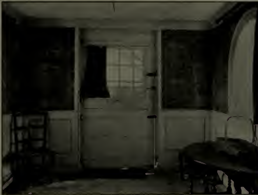
Inside the front door, which, with the tiled floor, is nearly as it was almost three centuries ago.
