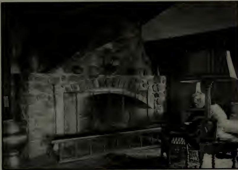
A happy solution of the corner fireplace problem, which necessitates an irregular shaped fire box and the location of the flue at one side
