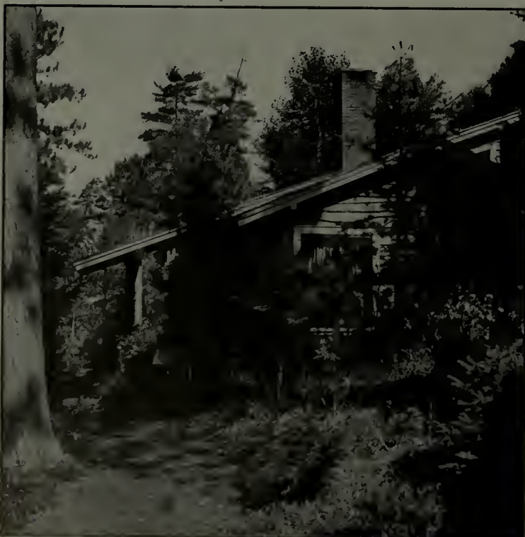
A new Adirondack type with a single-pitch roof. White Pine Camp, at Paul Smith's. Wm. G. Massarene, architect
