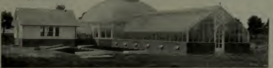
Rear View of Range of Greenhouses Just Completed on Estate of E. W. C. Arnold, Esq., Babylon, L. I. Front View Above
