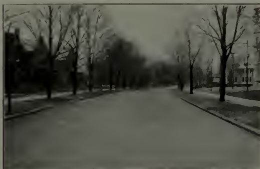
Bellflower Ave., Cleveland, O. Constructed with "Tarvia-X" in 1905. Note its present good condition after 10 years!
