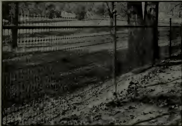
A 5-foot close mesh fence costing about $1.10 per foot, set
