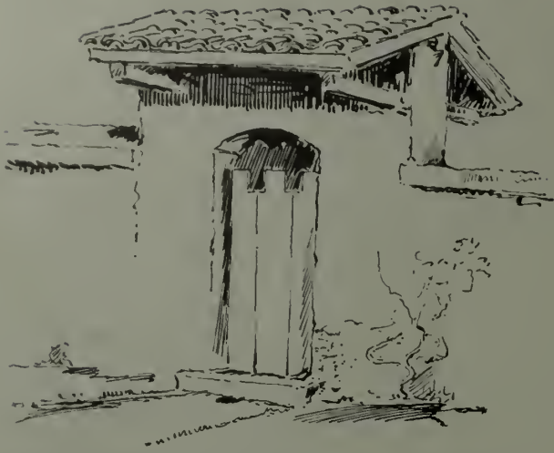
A sheltered gateway in a 'dobe wall—from Mexico. Two wooden beams are carried right through the wall to support the framework of rafters. Roughly made tile, such as the Mission Fathers used in Southern California, provide an enduring roof
