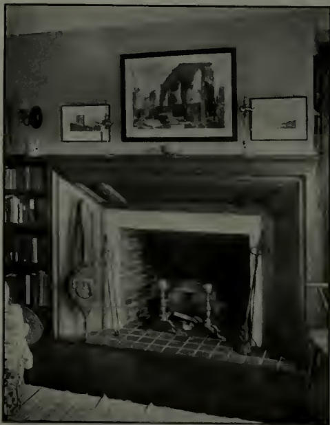
An unusual but attractive combination of marble facing with splayed paneled sides
