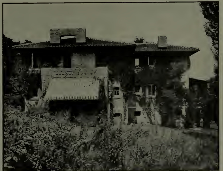
Tile inserts were used sparingly and in low tones, all tiles being handmade, of course. For the roof a Japanese pan tile is used, taking the run of the kiln in colors from smoky reds to salmon
