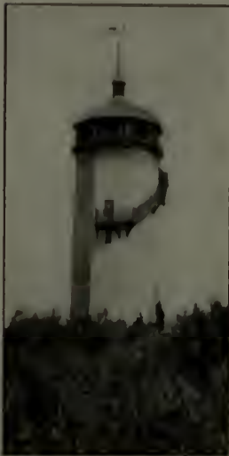
On the Mortimer Schill estate at Oyster Bay. At the bottom of the water tank the stairway leaves its shelter and winds aloft outside.
