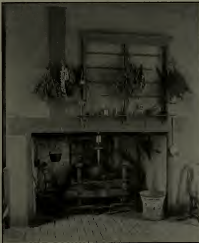
The most interesting feature of the great kitchen fireplace is the smoke-jack—a slender belt chain operating from a circular fan in the chimney that turns the spit. The chain runs over a flanged wheel at the end of the spit, and the draft from the fire keeps the fan in motion.
