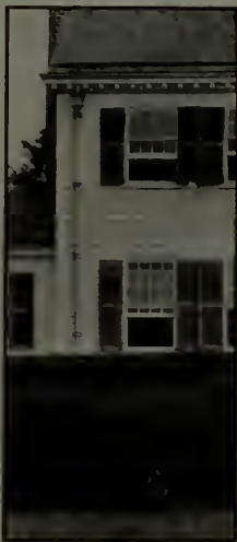
Circular-section leader with head, at Red Hill, the remodeled Patrick Henry house in Virginia
