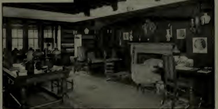
Showing beams stiffened by side casings, moldings covering what would in time become a crevice between plaster and beam. Fairacres, Jenkintown, Pa., Wilson Eyre, architect
