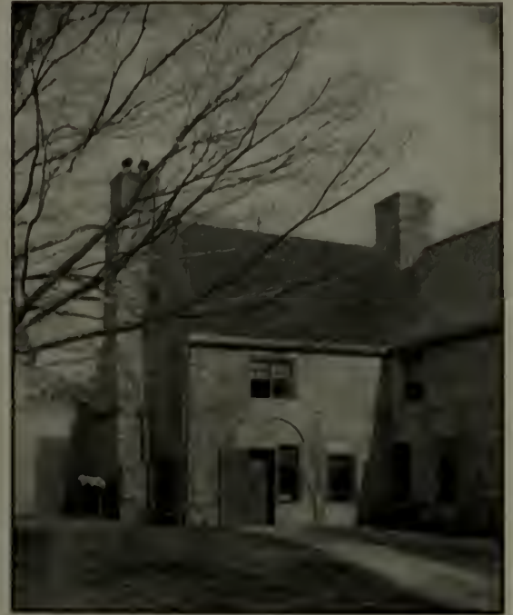
The rear wing upon the end of which the massive chimney indicates the great kitchen oven.
