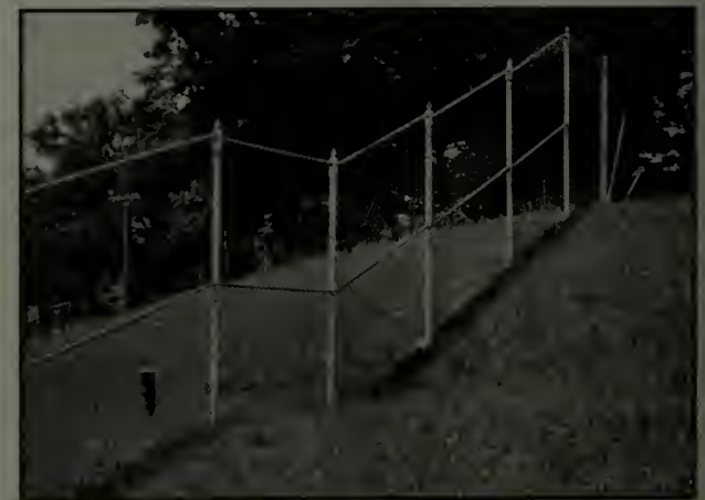
A 7-foot chain link fence without any frills, that will keep intruders at bay
