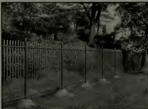
Iron picket and rail fence, the posts set in concrete, costing about $3 per foot
