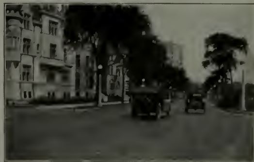
Lake Shore Drive, Chicago, Ill. Reconstructed with Tarvia in 1909. Heavy traffic but still good in 1915 as above.
