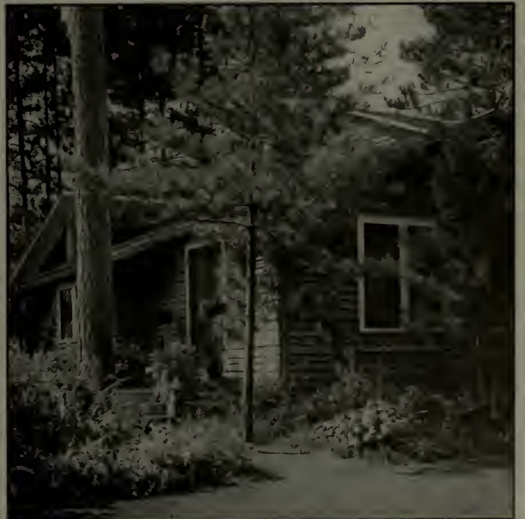
Another of the White Pine Camp group. The walls are of slabs sawed from the log and unplanned on the edges
