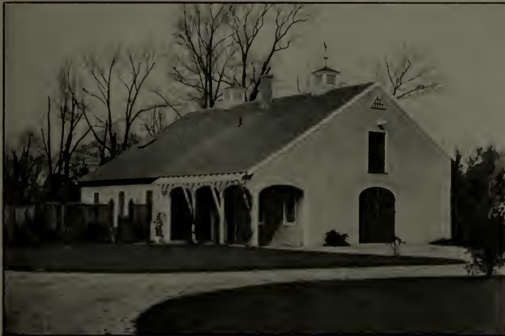
"Another stable . . . its wall finished in the Spanish texture of contrasting rough and smooth stucco." J. W. Ames, architect
