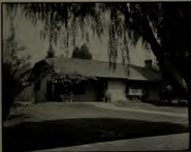
Stucco and shingles combined in a beautifully simple Pasadena bungalow. The wide overhang of the eaves belongs unmistakably to the buildings in this land of sunshine. Plan above
