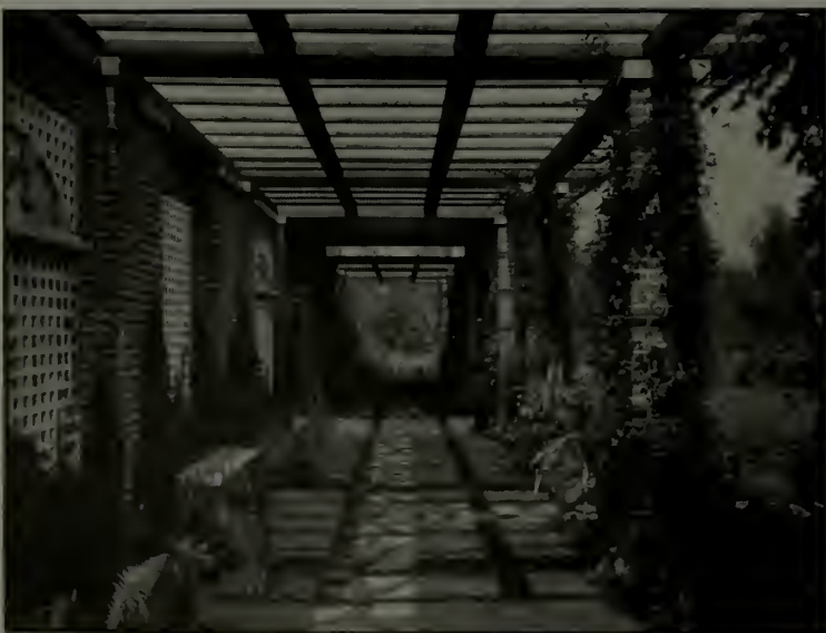
An arbor screen bounds one side of the garden, affording an architectural line of enclosure and a retreat from which to view its broad pattern
