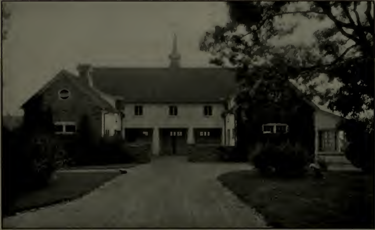
Philadelphia in inspiration, with heavy white tapering pillars and overhanging upper story facing the barn-yard." This is the combined stable and garage of the Steel house shown on pages 50 and 51. Percy Ash, architect
