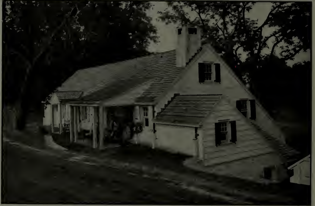
Cottage of roughcast and whitewashed stone on Philander C. Knox's estate at Valley Forge, Pa. Duhring, Okie & Ziegler, architects
