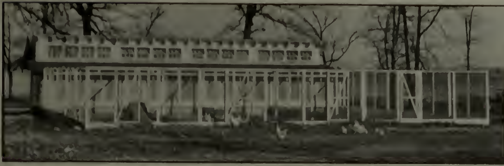
Model poultry house at Edellyn Farm, the country home of Mr. Thomas F. Wilson, Waukegan, Ill. It is of the semi monitor type, and is a good example of just how attractive such a building can be made if one goes about it in the right way. George F. Dippell, architect.
