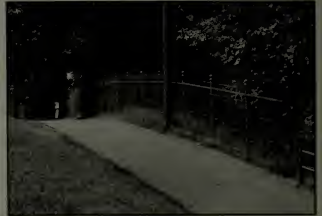
A 6-foot unclimbable fence with barbed wires carried on steel arms
