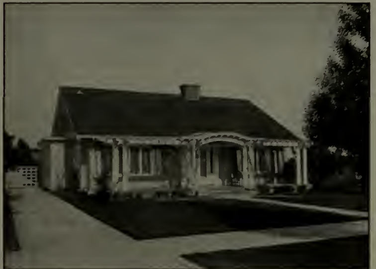
A very simple clapboarded bungalow that has distinction by reason of its pergola porch. Plan at left
