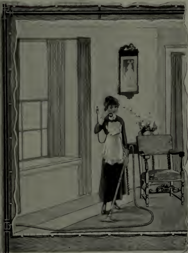
This illustration shows the baseboard outlet for the vacuum cleaner. The cleaning hose can be carried from room to room.
