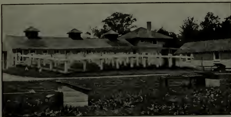
Rear view of same brooder house, showing the outside covered yards. In the foreground are individual brood coops with wire runs. Alfred Hopkins, architect.
