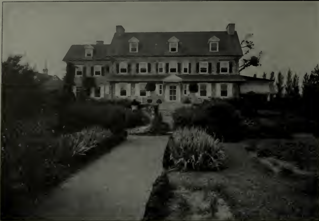
The garden front of Windham. In keeping with the traditions of Philadelphia and its suburbs is the characteristic Germantown hood over the first story windows
