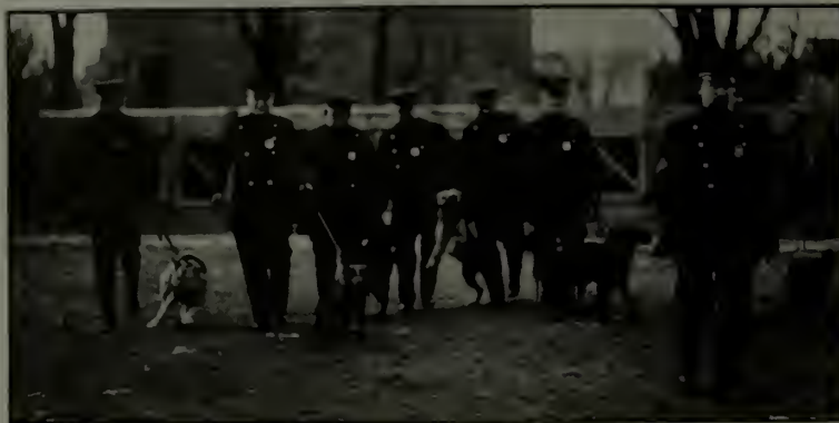
The Parkville squad mobilizing. The new kennels are in the background
