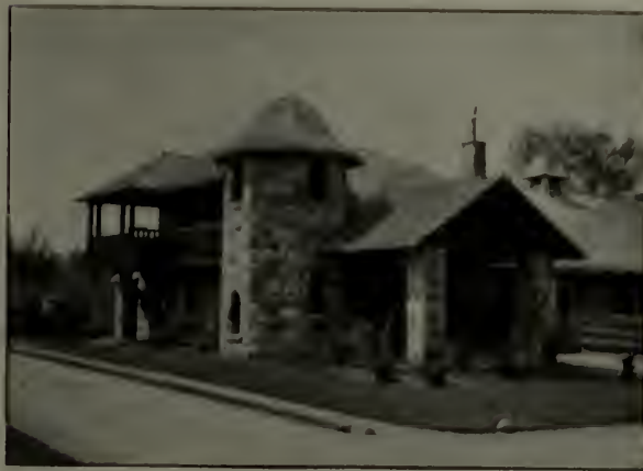
The tower in Mr. Harry Fisher's stables at Greenwich, Conn., provides a stairway from the first floor to the men's living quarters above.
