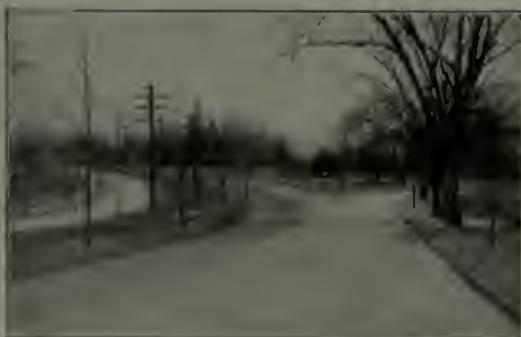
Newton Boulevard, Newton, Mass. Treated with "Tarvia-A" nine years ago. Still in good condition.
