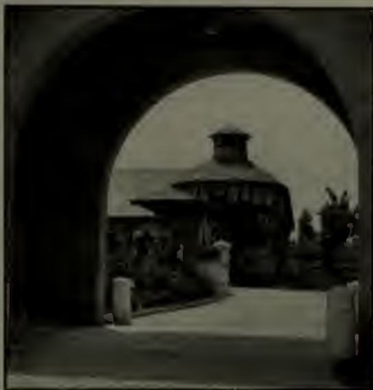
Another tower on the Schill estate, providing a wash room below for the men, and space for the birds above.
