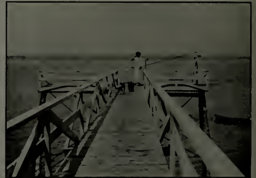
The floor of the T-shaped pier is well above the highest sea
