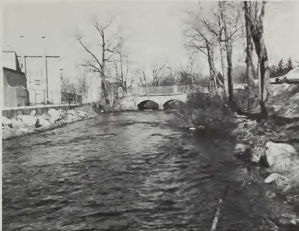
Ashland -- This twin stone arch bridge, near the General Electric Telechron Plant, is one of four restrictive stream crossings on the Sudbury River. (SCS photo)
