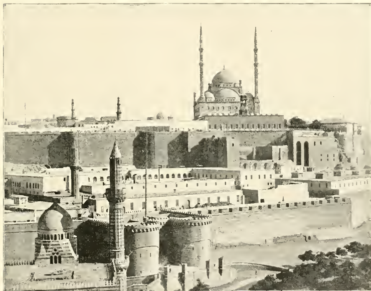
Gate of the Citadel, Cairo.
