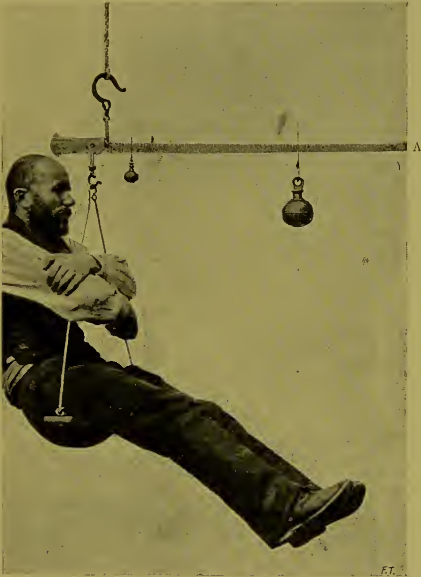
FIG. 62.—Roman balance made use of on the Monte Rosa expedition.
