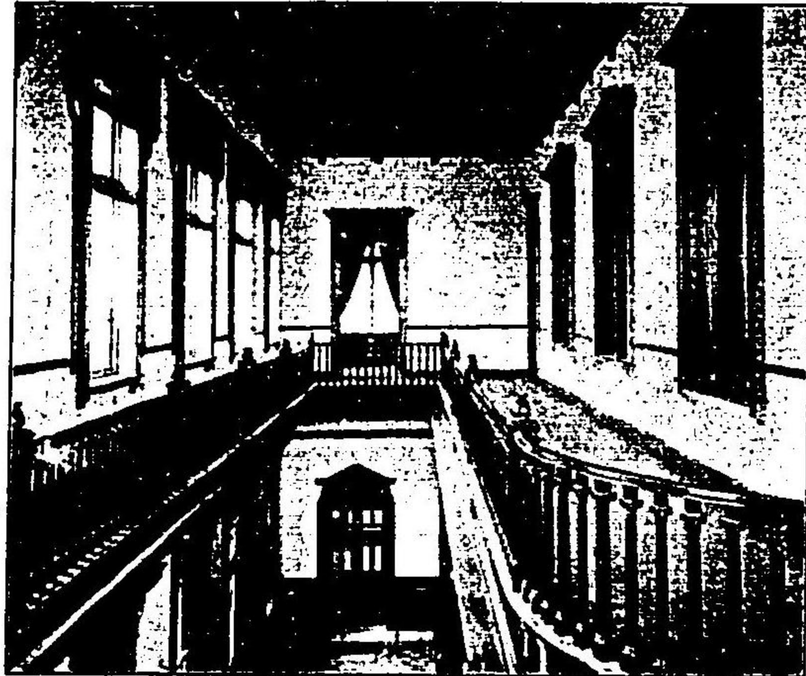
Interior View of Tokyo Bank.
