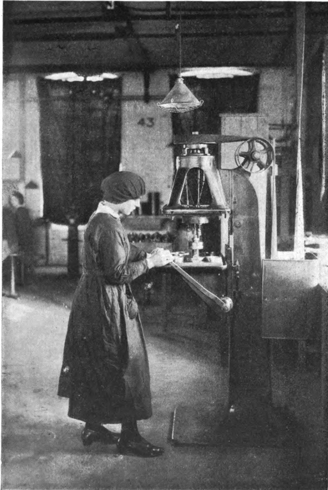
Drilling small parts (of ball bearings) with multiple spindle drill.
