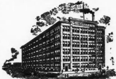
FACTORY 132 ND TO 133 RD ST & BROOK AVE
