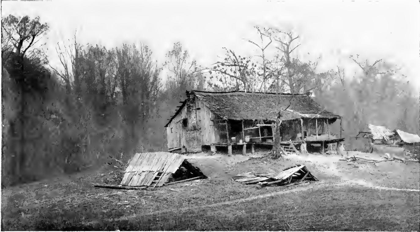
FIG. 13.—House on mound at Shadyside Landing, Miss., showing part of mound under the house, protected from wash of rain, and illustrating the erosion to which mounds sometimes are subjected.
