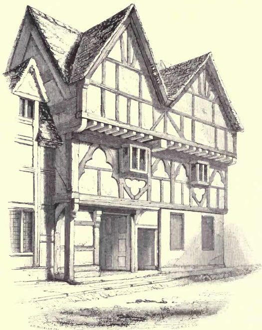
TIMBER HOUSE AT TAMWORTH.
