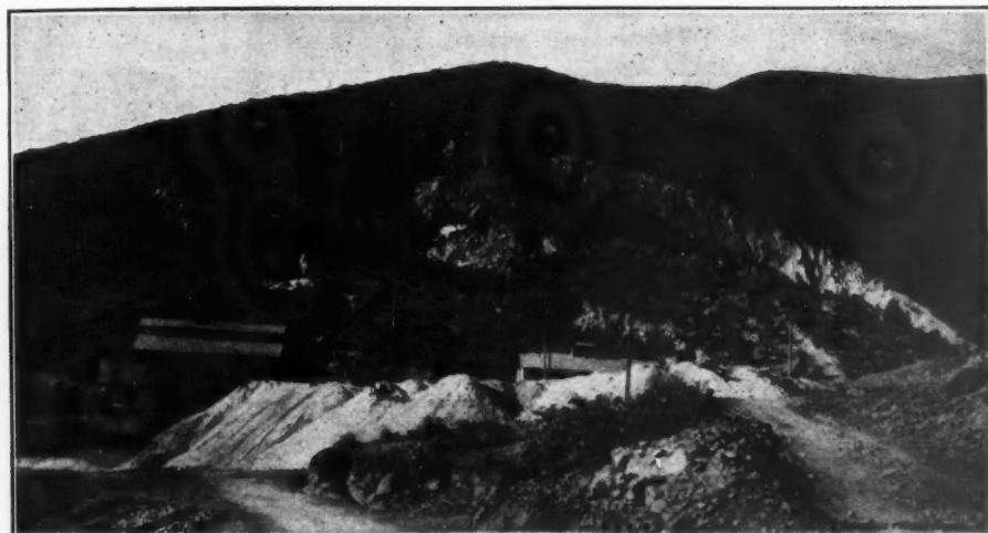
VETA GRANDE MINE, CANANEA, SHOWING CAVED GROUND
