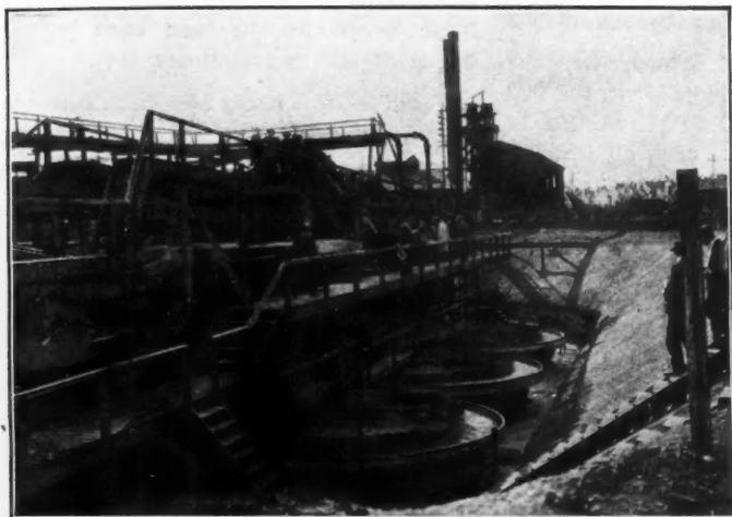
CALDECOTT SAND TABLES AND CONE CLASSIFIERS AT SIMMER & JACK MINE, SOUTH AFRICA
