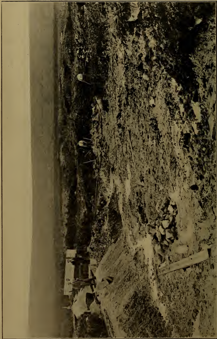
Fig. 2.—Stream-tin workings in Kenton Marsh, north-west of Buttern Hill (Cornwall).
