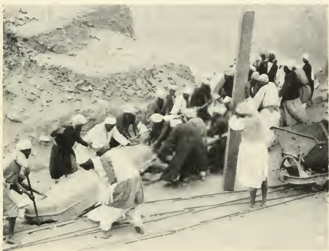
FIG. 17. HAULING LINTEL OF MAIN DOORWAY
