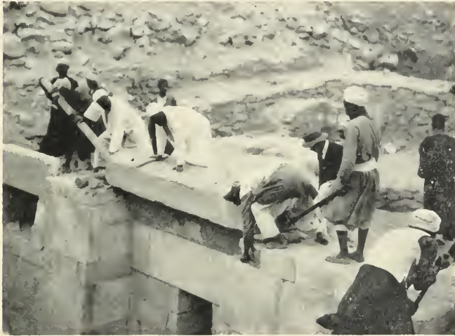
FIG. 16. REMOVING LINTEL OF MAIN DOORWAY
