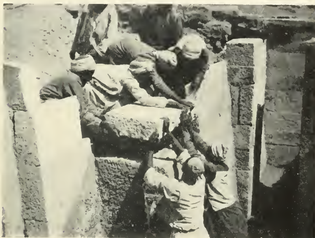
FIG. 20. REMOVING BLOCKS FROM FAÇADE
