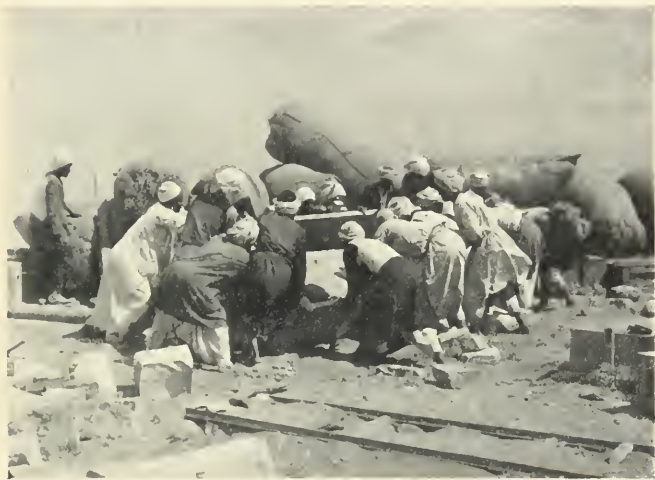
FIG. 18. PACKING LINTEL OF MAIN DOORWAY
