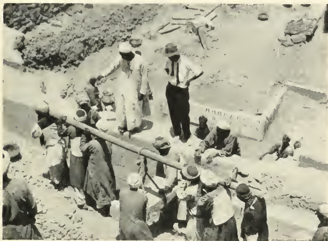
FIG. 23. METHOD OF CARRYING BLOCKS
