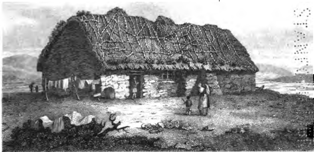
A Cottage in Italy.
