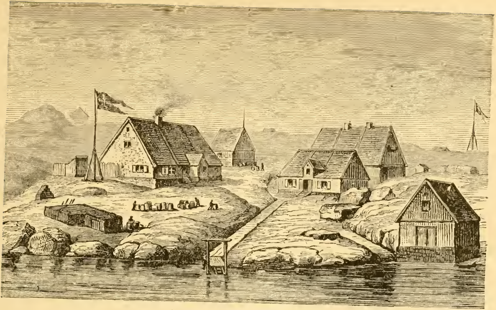
A VILLAGE IN GREENLAND.
