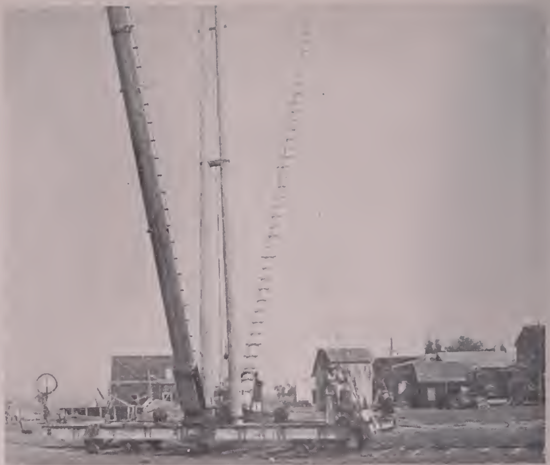
Right: Close view of RKO's new camera-boom; note pneumatic winches, generator for camera-driving current, and rigidly-braced construction. Below: The boom in use; at bottom: dropping miniature bombs.
