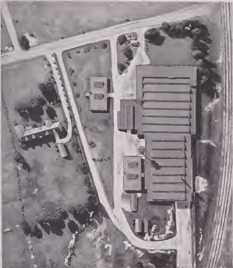
NOW YOU SEE IT. Before the camouflage experts went to work, this factory—a model, for test purposes—was photographed from the air on conventional panchromatic film. The bomber's eye would see what you see—a perfect set-up for destruction.
