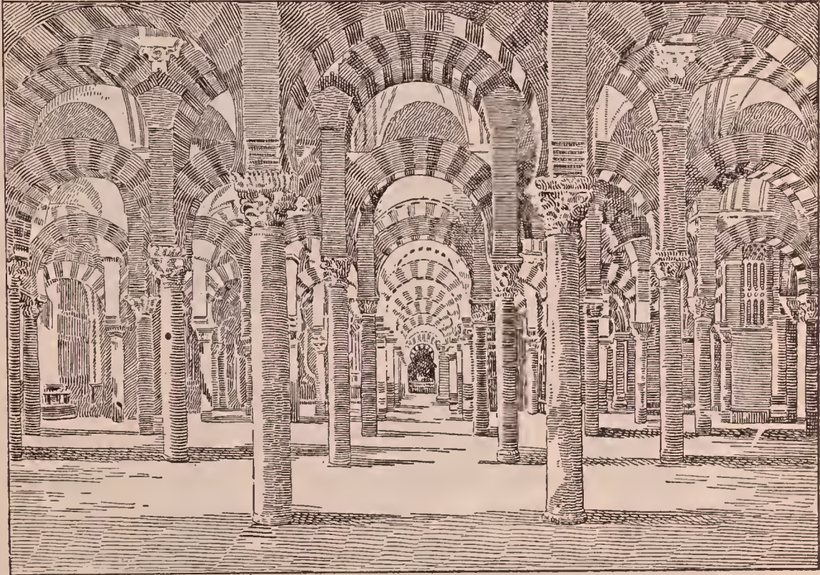
INTERIOR OF THE GREAT MOSQUE OF CORDOVA
