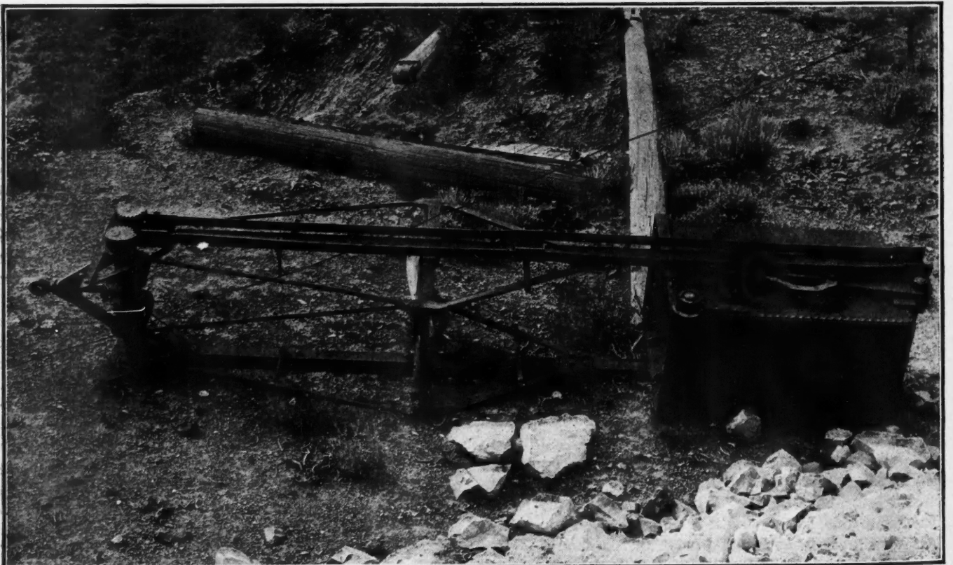
ONE OF THE EARLIEST COMBINATIONS OF CAGE AND SKIP USED IN VERTICAL SHAFT ON THE COMSTOCK
