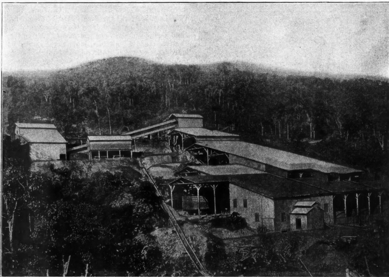
MILL AND CYANIDE PLANT, EDEN MINE
