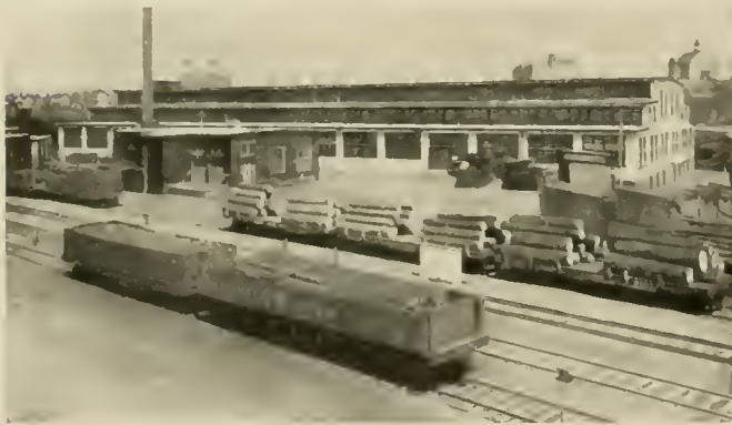
Rear of Main Plant
