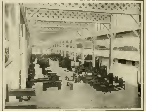
Erecting Floor Main Building
