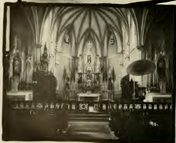
INTERIOR ST. ANDREWS R. C. CATHEDRAL
