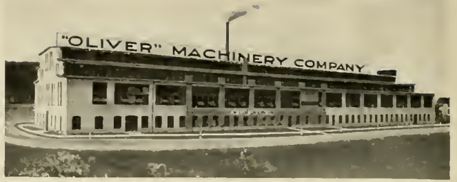
Main Plant—Corner Goldbrook and Clancy Streets
