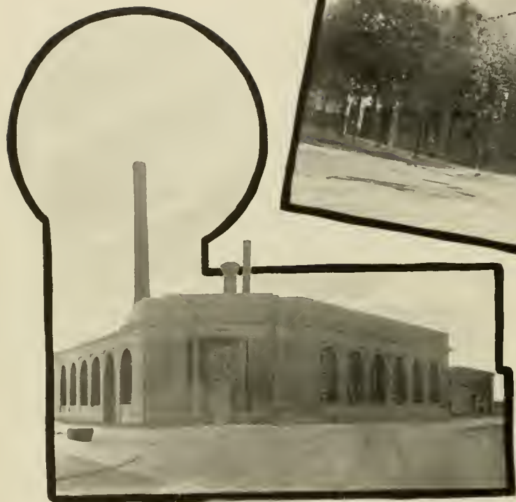
NEW PUMPING STATION
