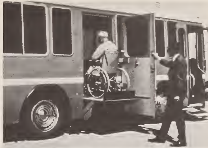
These photos illustrate special bus modifications used to assist handicapped riders, including a hydraulic ramp to raise wheelchairs to floor height and a special low-step design with extra step extension to aid ambulatory users.
