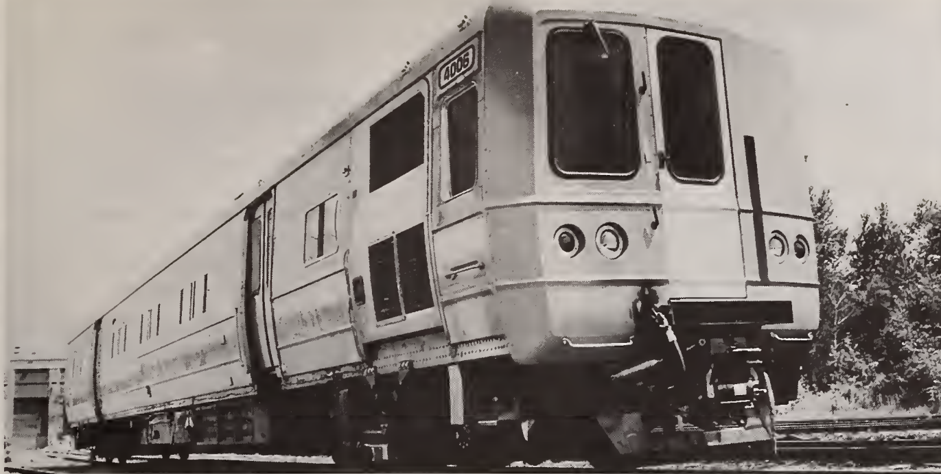
General Electric's Gas Turbine/Electric commuter rail cars are fitted with engine units that swing out for maintenance.
