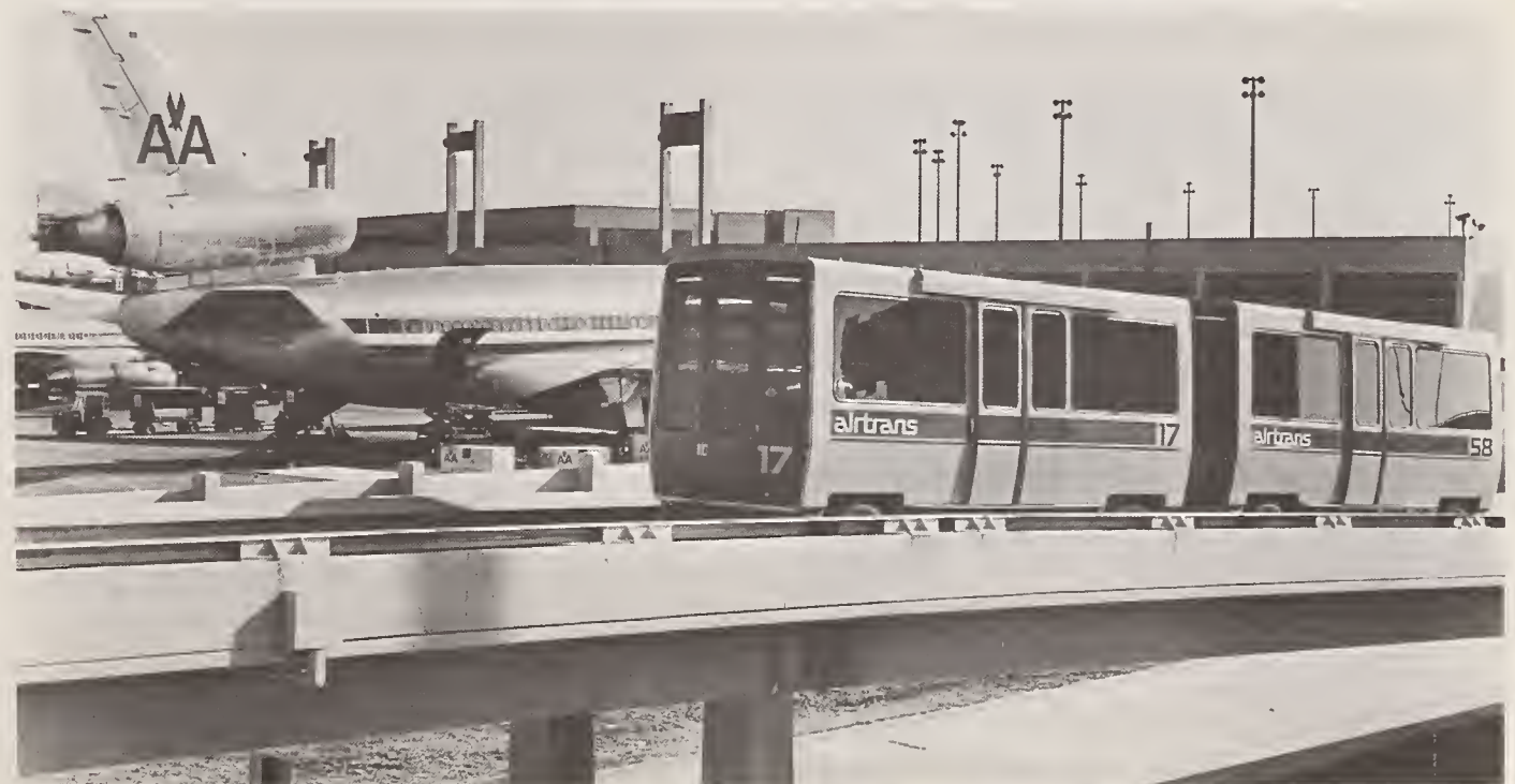
The AIRTRANS system at the Dallas/Ft. Worth Airport is being assessed to provide data that will aid planning and implementation of future automated guideway systems.
