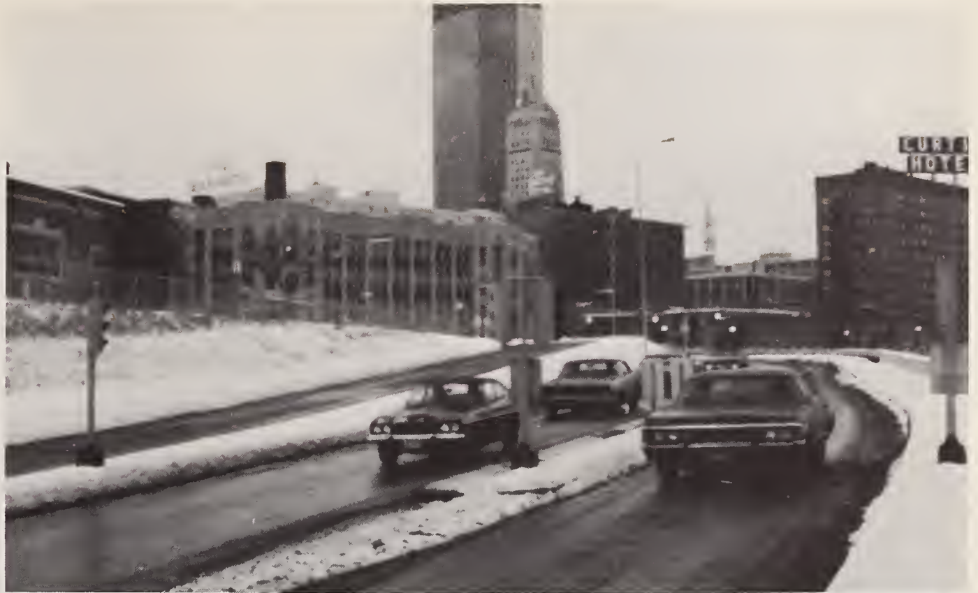
Metered freeway ramps combined with bus signal preemption controls are expected to speed traffic flow in Minneapolis (I-35W).
