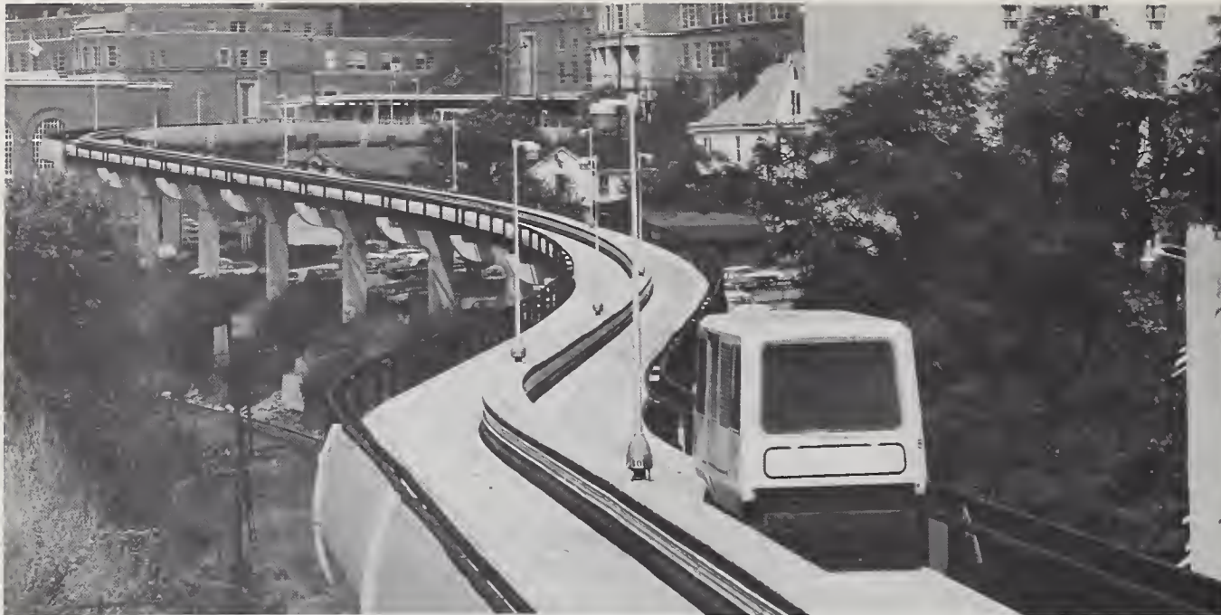
The Morgantown PRT system links distant reaches of the West Virginia University campus by elevated automated guideways.
