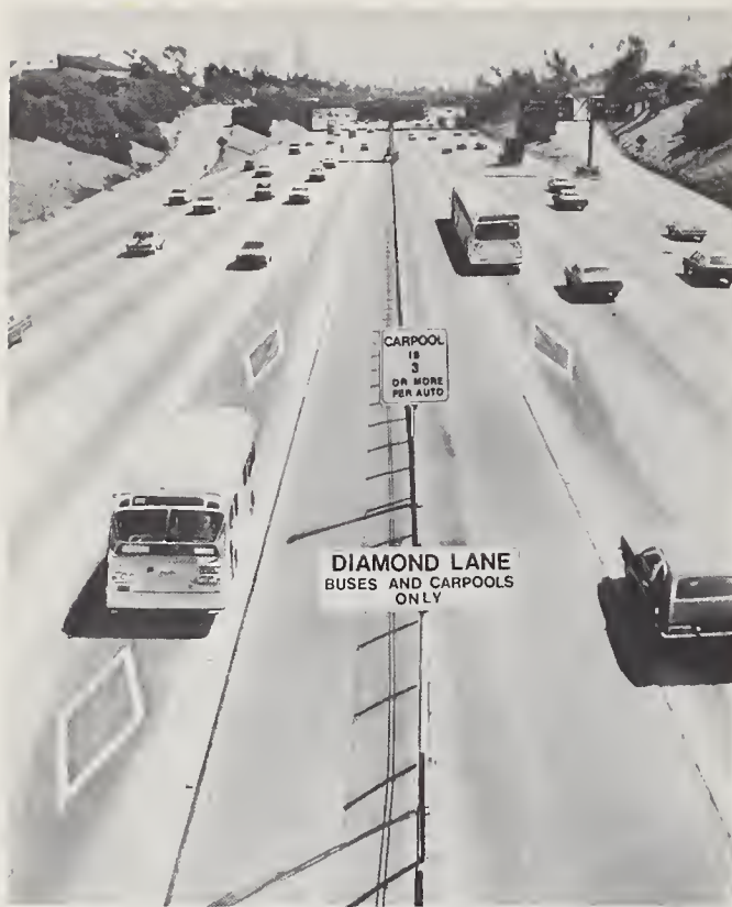
"Diamond Lanes" provide non-separated bus and carpool lanes on the Santa Monica Freeway near Los Angeles, California.
