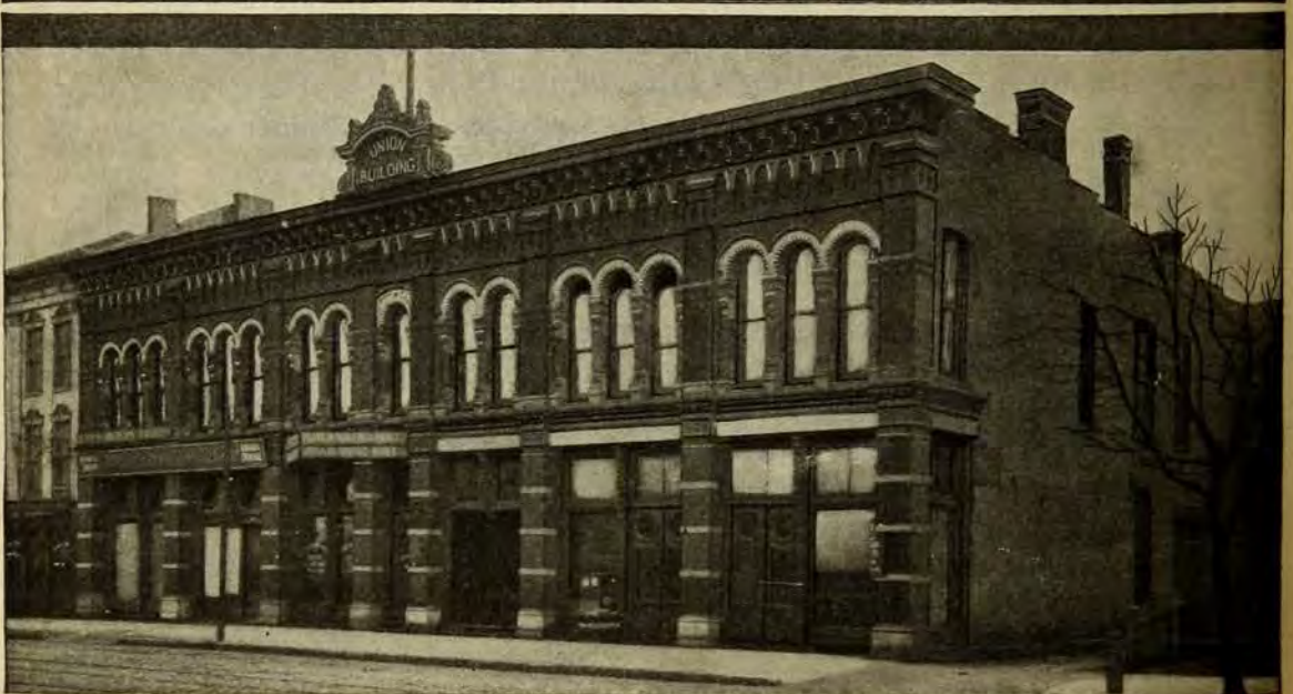
UNION BUILDING, INDIANAPOLIS, INDIANA, ROOFED OVER 20 YEARS AGO.
