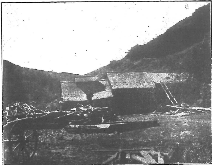
B. Typical Country Salt Plant, 8 Miles East of Nephi, Juab County, Utah. The Brine is Evaporated in Small Open Pans.
